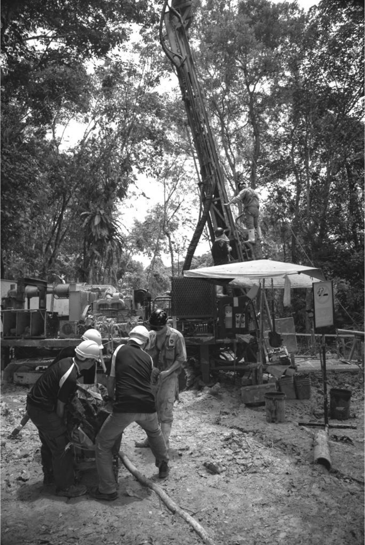
Exploration Drilling - Bau Gold Field, Malaysia
