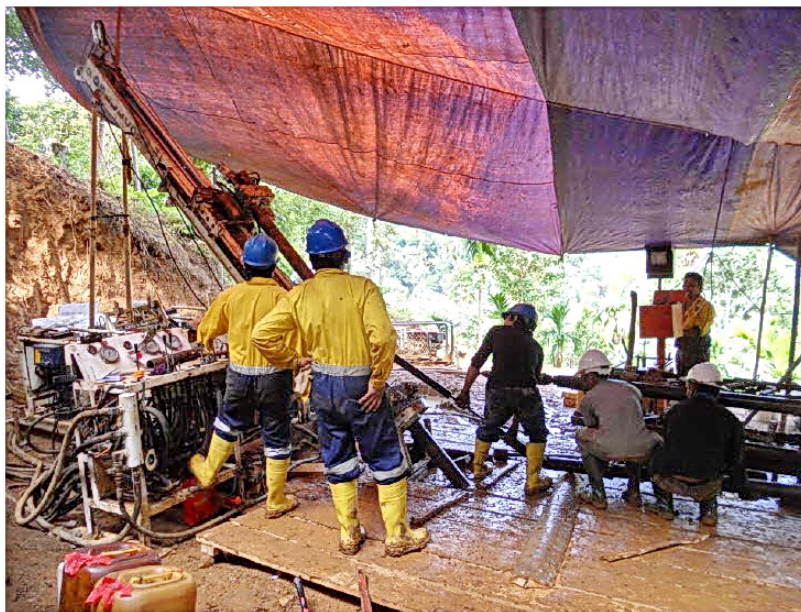
Figure 3: Commencement of drilling at site of PMD001
