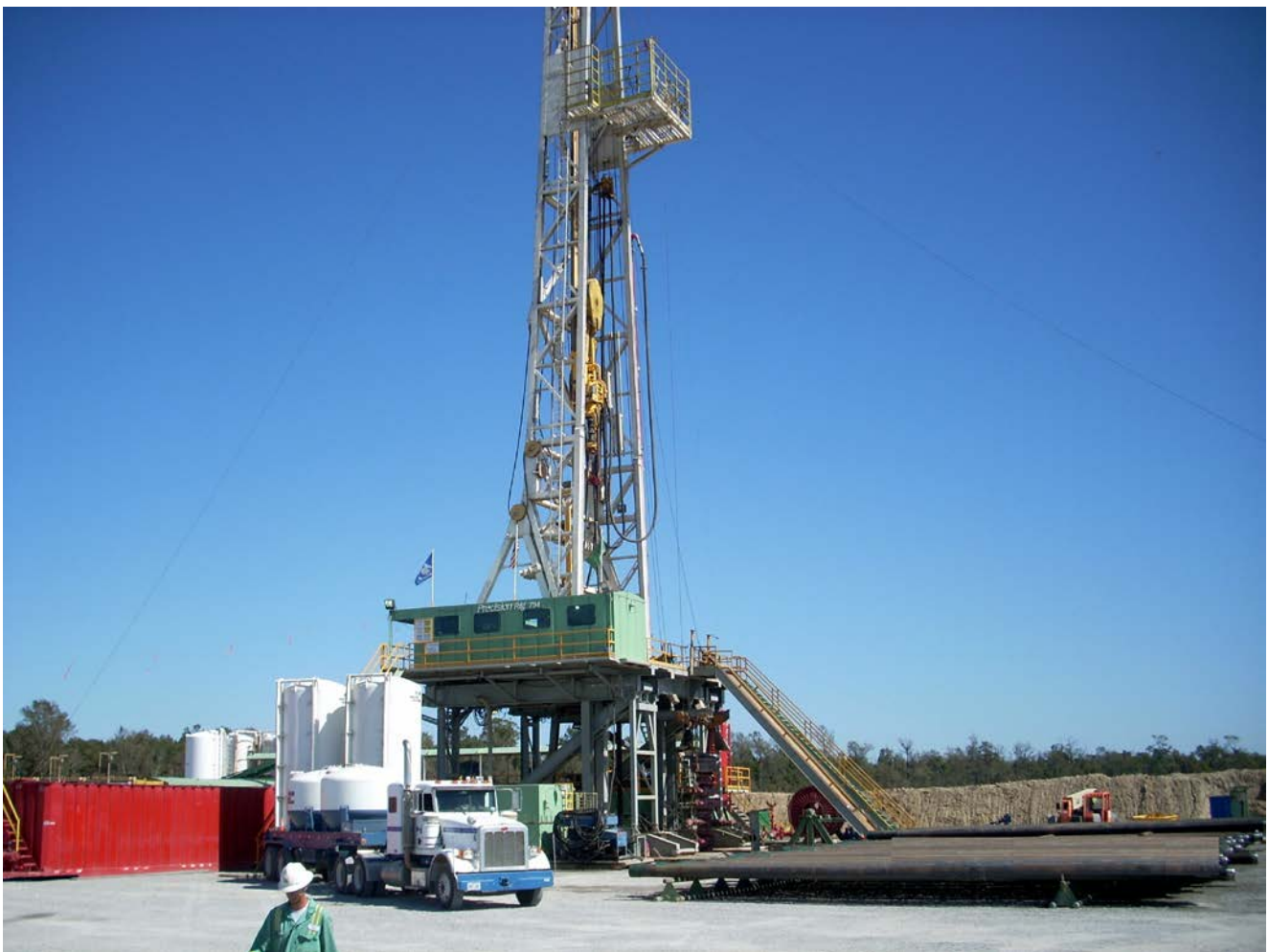
Drilling begins on the Rosewood plantation 21H well
