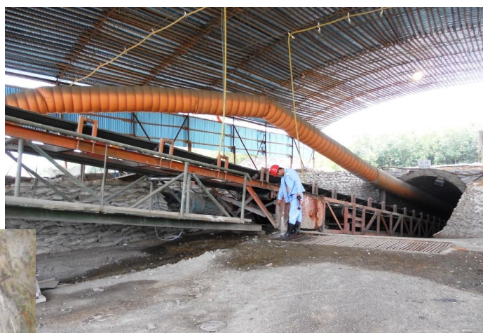
Above: Main Entry and Coal Conveyor
