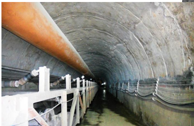
Above: Main Entry with Shotcrete Lining
