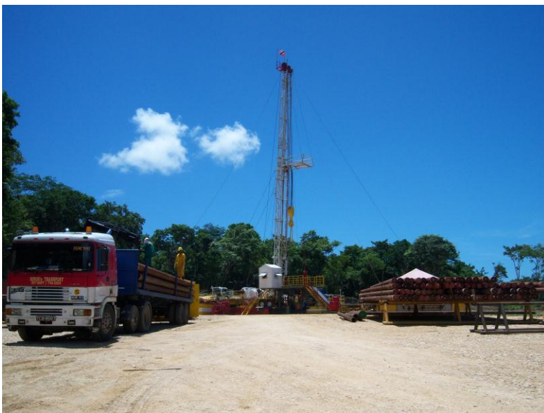
Figure 3 – Drilling Rig on Location
