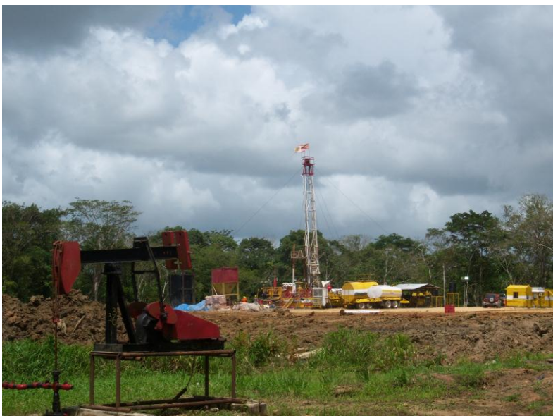
Figure 4 – Drilling Rig on Location
