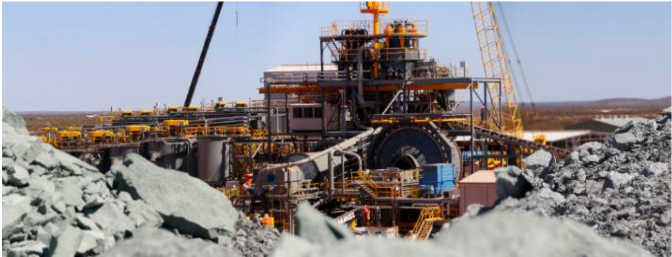
Grinding and Flotation areas – view from ROM pad
