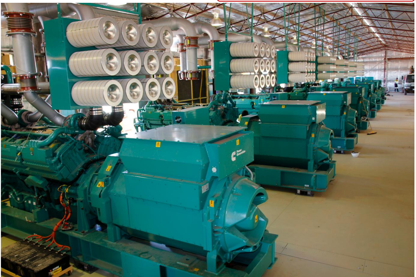
Completing installation of 2MW Generators
