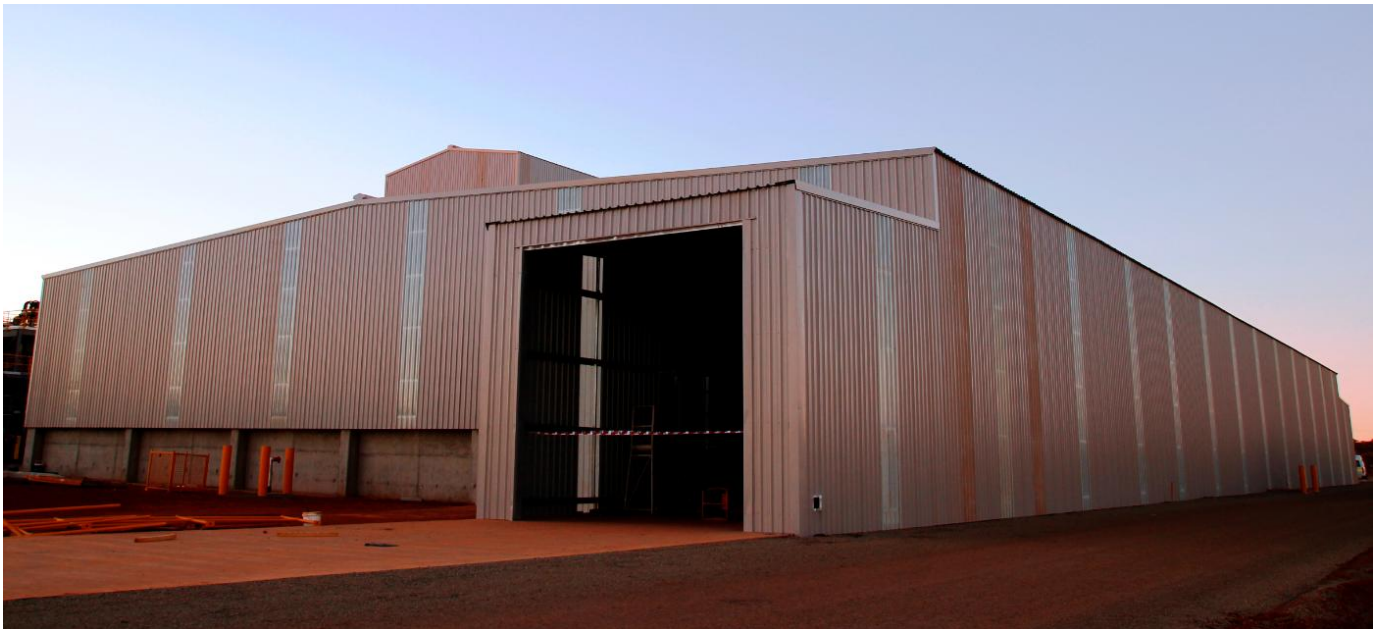
Concentrate shed – nearing completion
