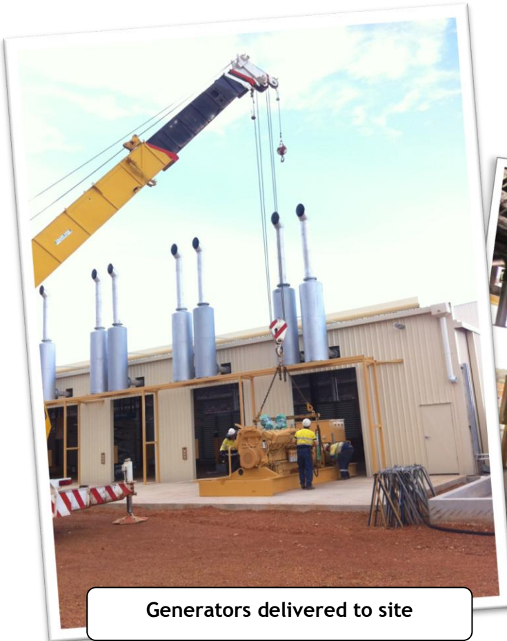
Power House ready for the installation of Gensets
