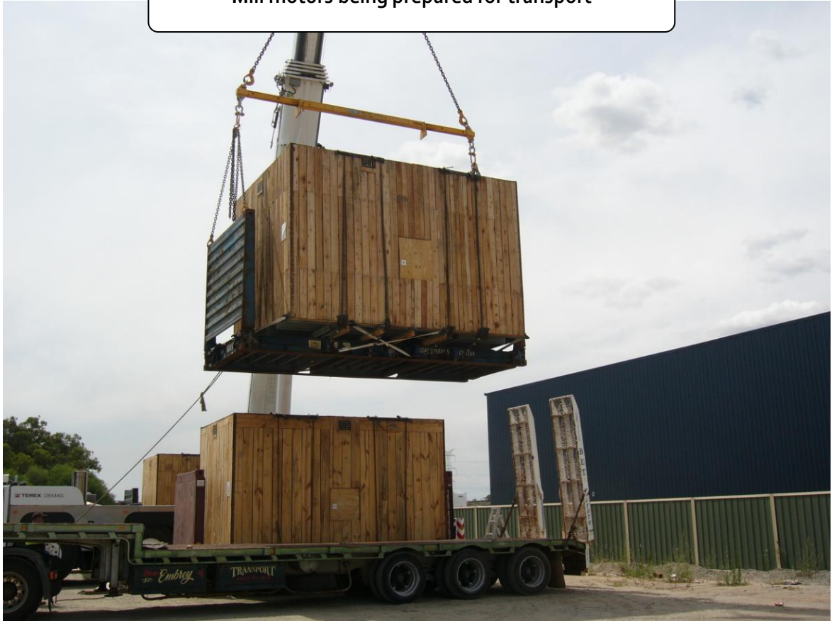
Mill motors being prepared for transport
