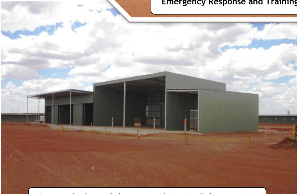
Heavy vehicle workshop - completion in February 2012
