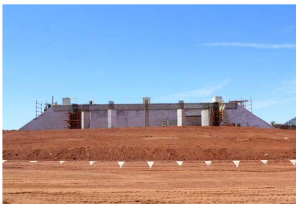
Figure 7: Fine ore bin tunnel
