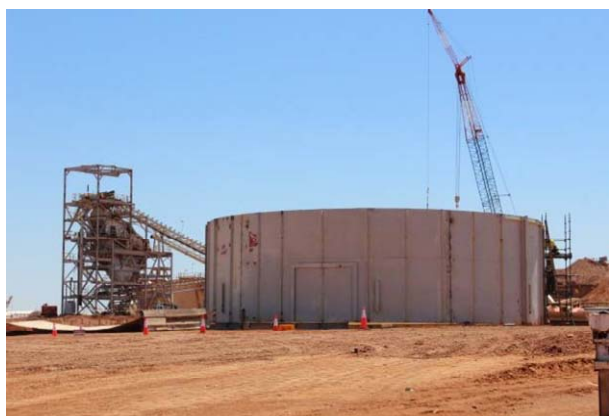
Fine ore bin construction
