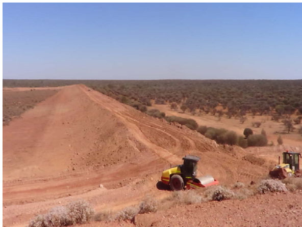
Figure 9: Tailings dam lift under construction
