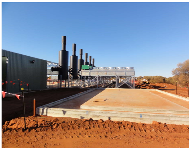
Figure 6: Power plant construction
