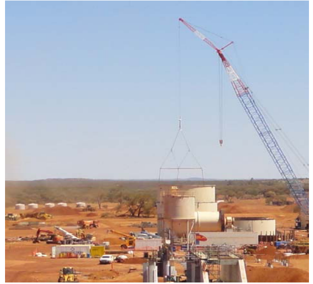
CIL tank construction
