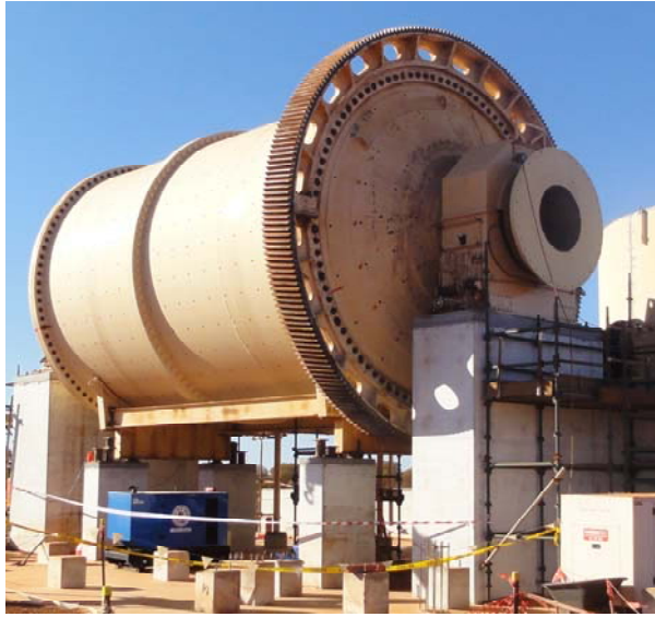
Figure 8: Ball mill installed on plinths
