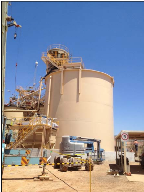
Figure 4: Photo of Lakewood Gold Processing Facility upgraded circuit showing new 150 cubic metre leach tank, materials handling system with 1.6 megawatt ball mill in the background.
