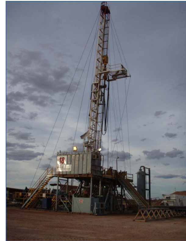
Ensign 918 drilling Marsden 1
