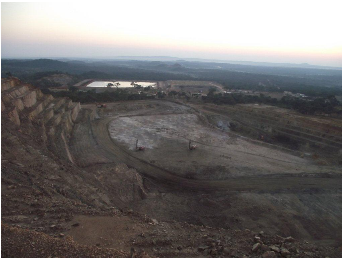
Kipoi Central open cut mine
