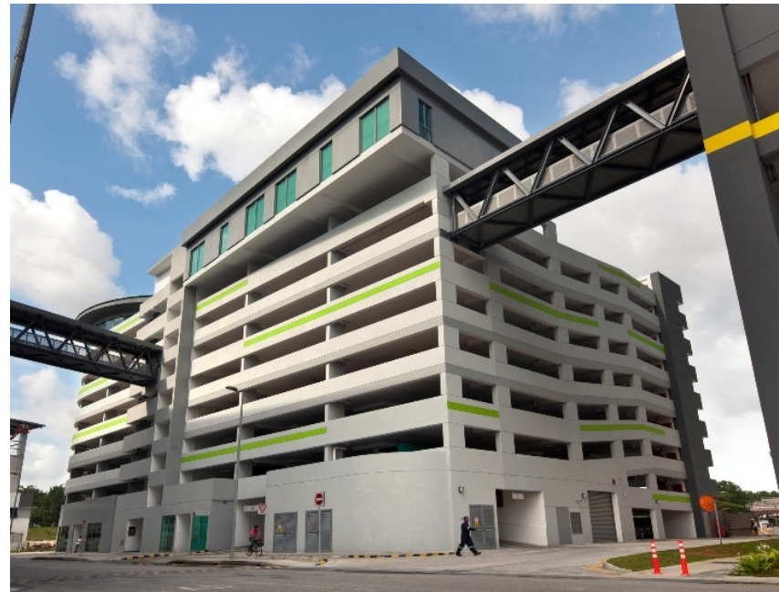
Multi Storey Car Park
