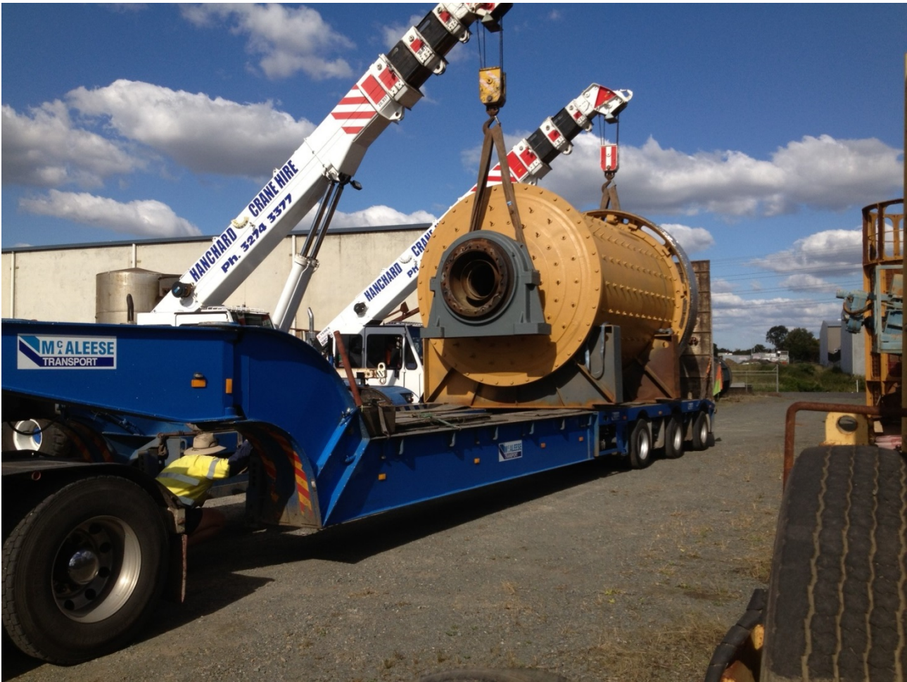
Figure 2. Off-site refurbishment of Ball Mill (pictured) nearing completion at Index Industrial in Brisbane.
