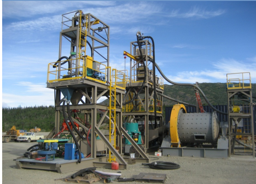
Example of a gravity gold plant with ball mill and Knelson concentrator. Image source: www.knelsongravitiesolutions.com
