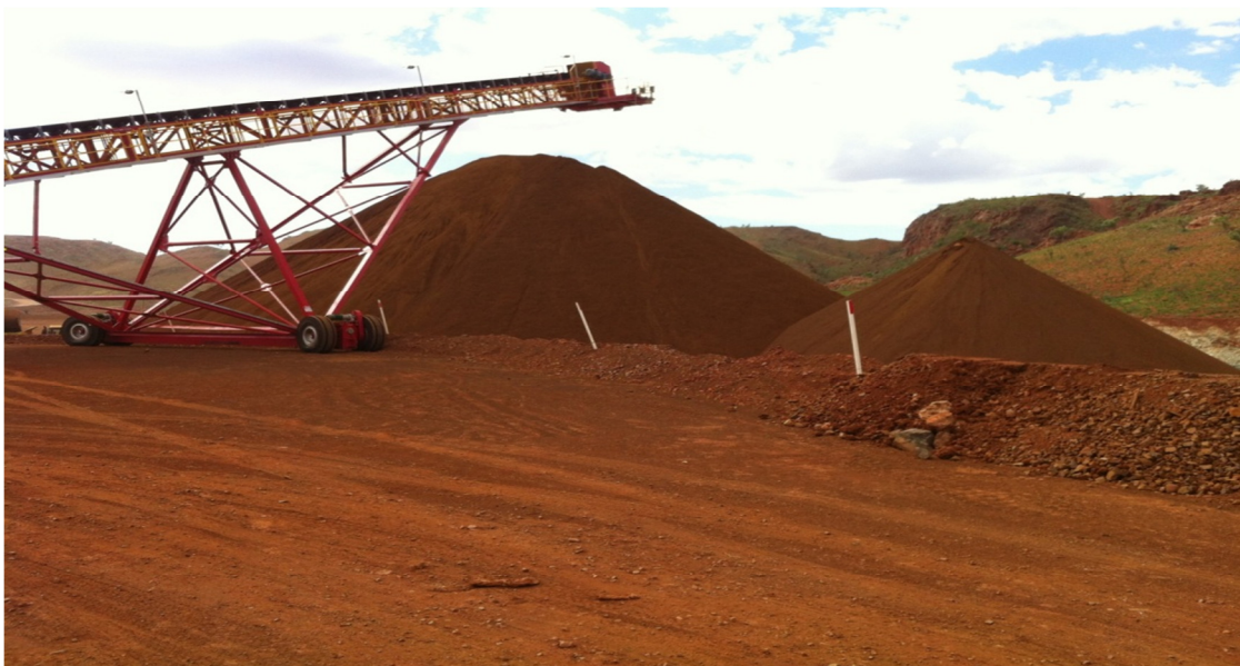
First Crushed Ore at Abydos
