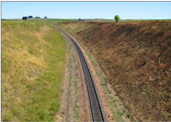
Railway runs through the project
