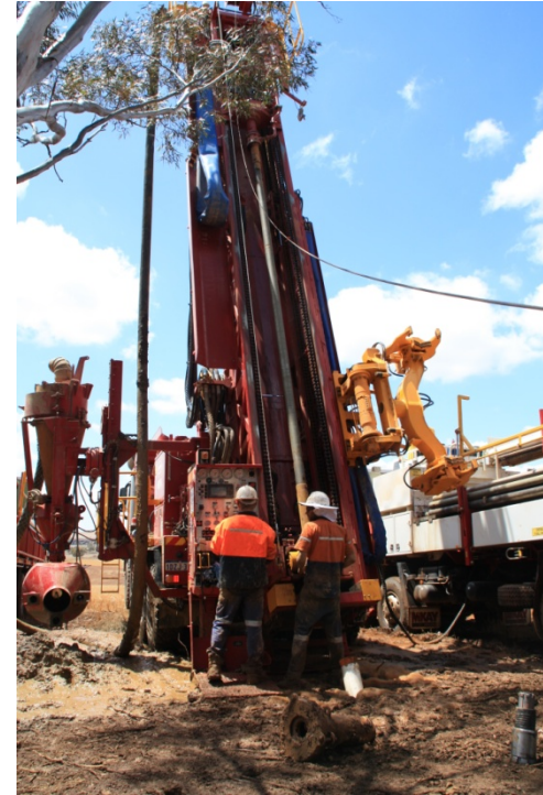
First phase RC drilling at Pingaring Nickel Project, Western Australia
