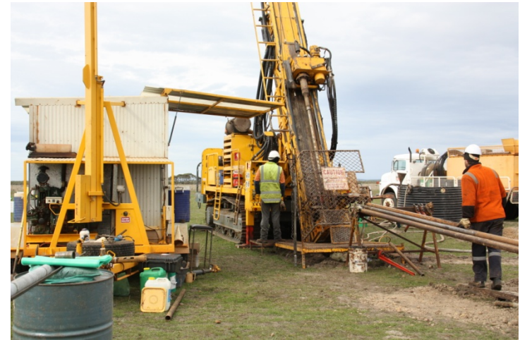
Stage 1 diamond drilling at Southdown Extension Iron Ore Project, Western Australia
