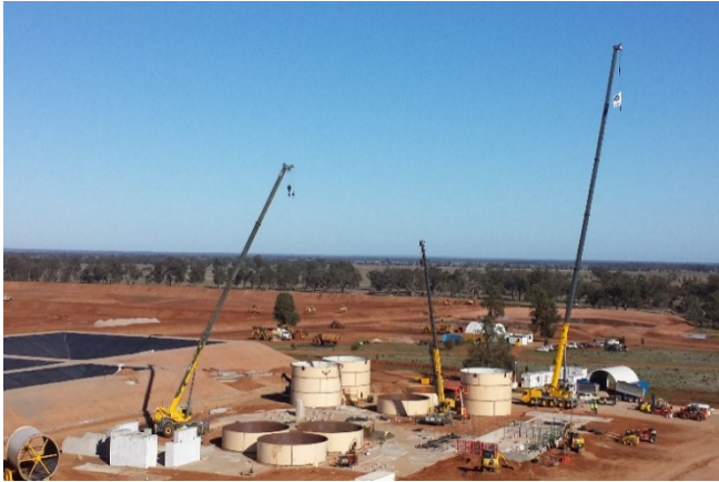
Central CIL plant construction
