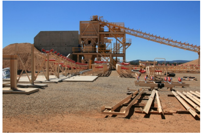
Ore bin and ROM pad
