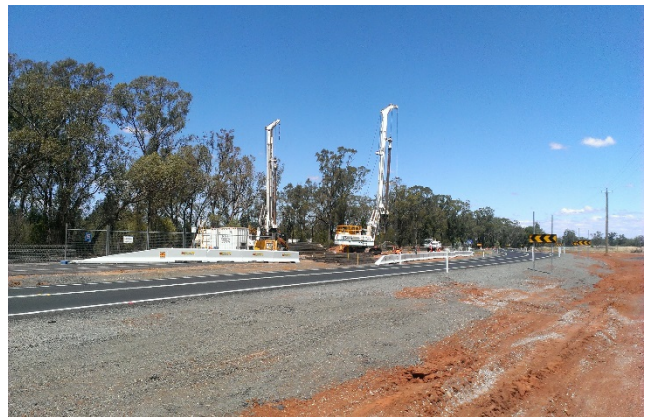
Piling works for Newell Highway underpass
