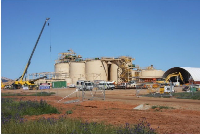
CIL plant construction
