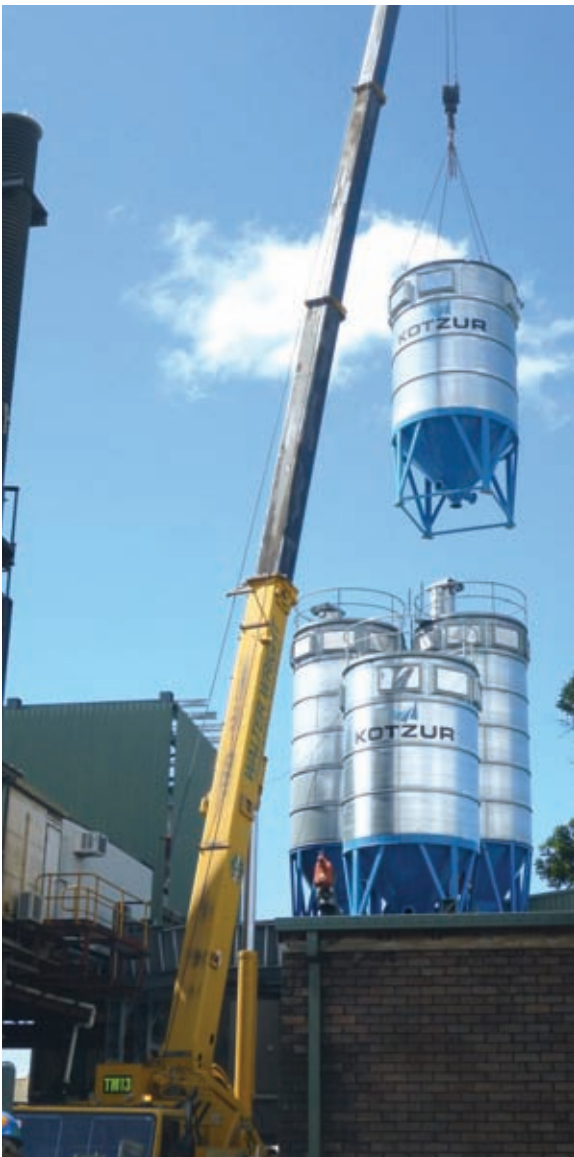
Installing the silo for the reduced iron product
