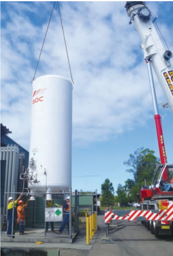
Installing a larger nitrogen storage tank
