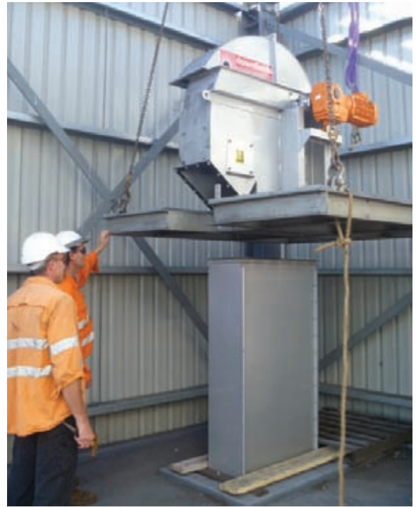
Installing the drive head of the bucket elevator used to transfer the briquetted iron product
