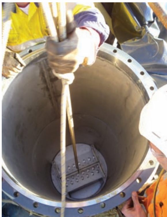
Installing the trays into the columns
