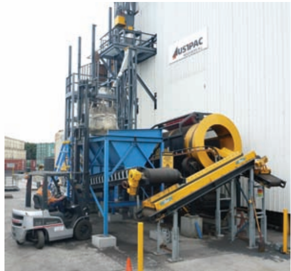
Charging the mill scale hopper
