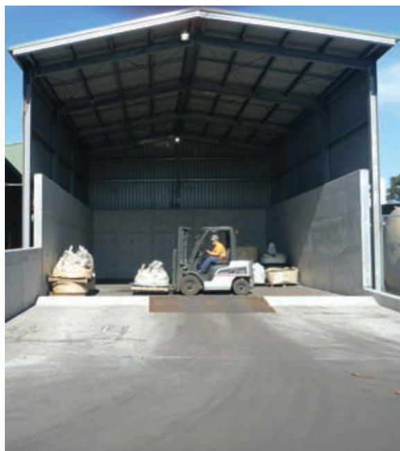
Banded bulk mill scale storage ready for first delivery
