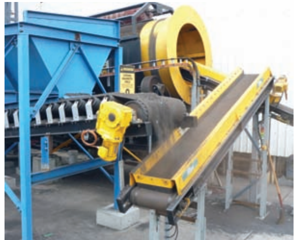
First feed from the mill scale hopper
