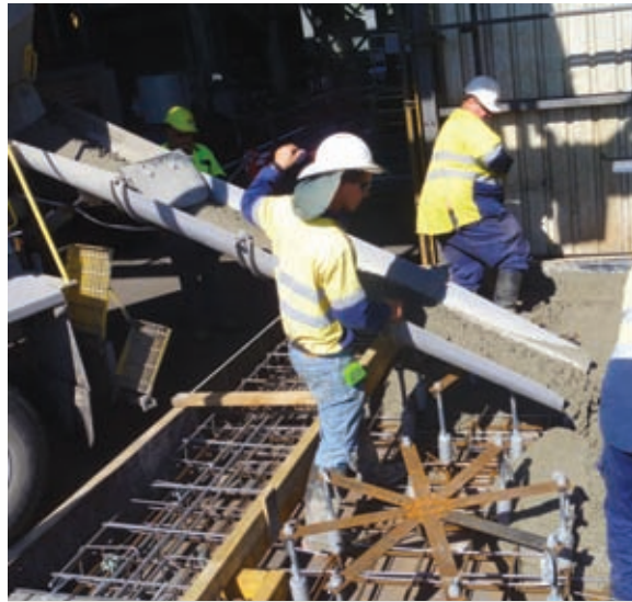
Pouring foundations for the CO 2 stripping and absorption columns
