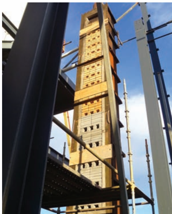
View of a stove packed with refractory bricks prior to installation of the front cover
