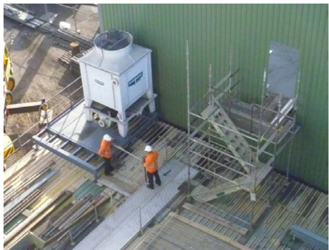
Cooling tower installed beside temporary access stairs to the plant room
