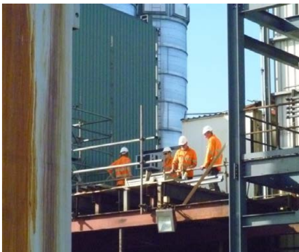
Installation of scaffolding for access from the control room
