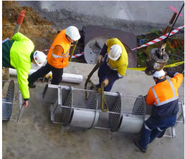
Preparing the internal stainless steel trays for hoisting. The trays facilitate gas-liquid contact and achieve gas absorption in the columns
