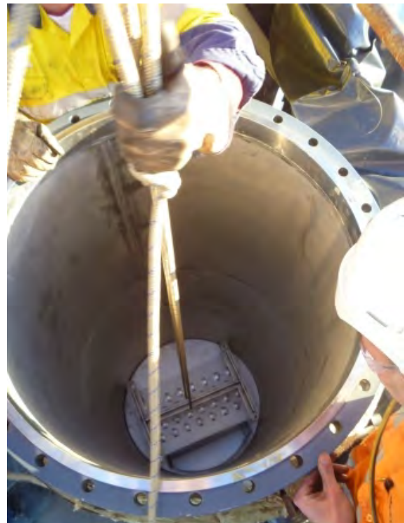
Installing the trays into the columns
