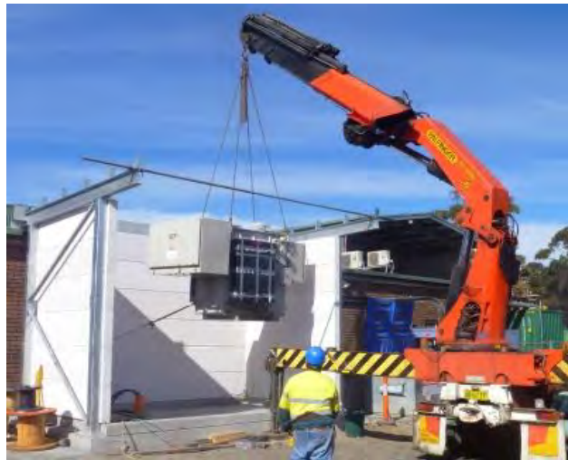
Installing the high voltage transformer
