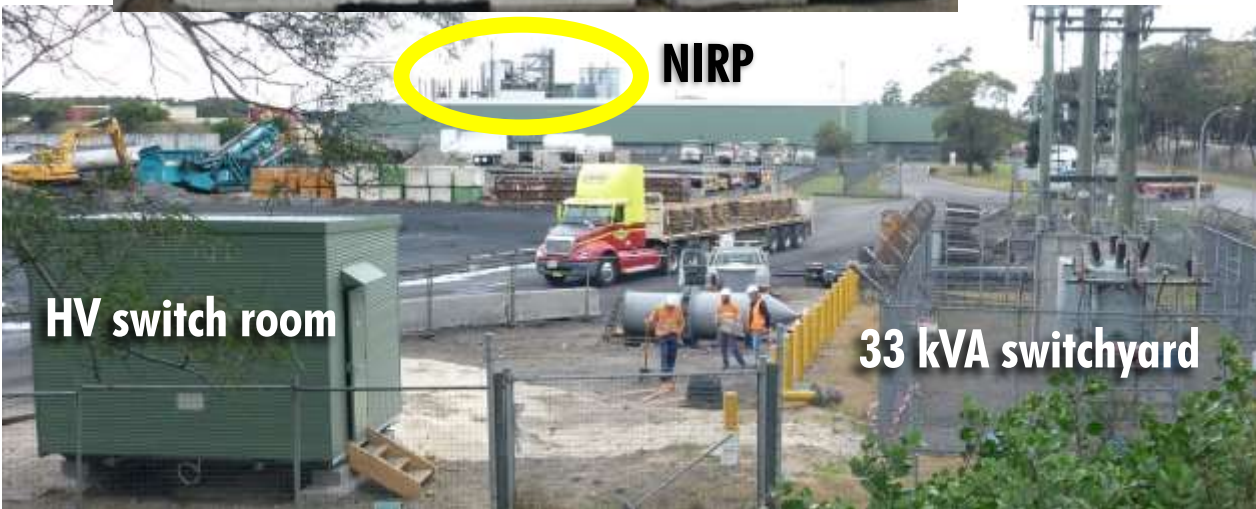
Drawing HV cable from the transformer to the switch room
