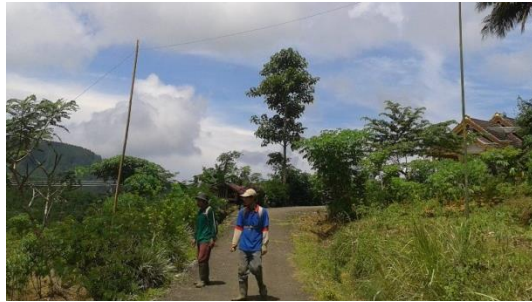
Line crossing above the main road
