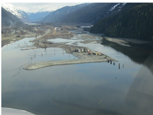
Stewart World Port dock under construction
