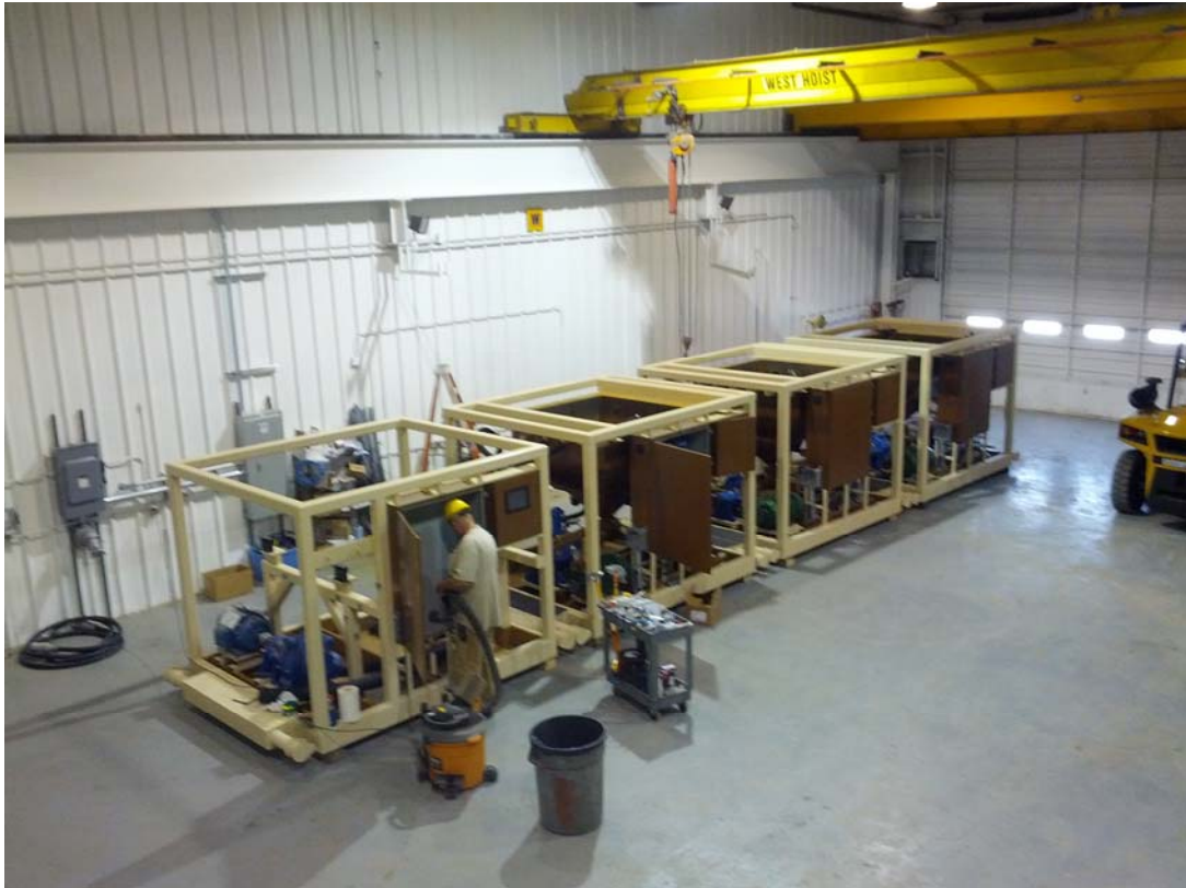
Assembly and integration of the 5th Unit in advance of initial tests with mineralised material.
