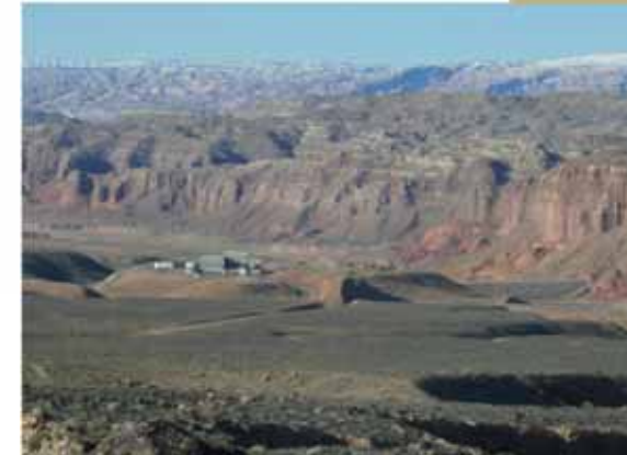
Shootaring Mill with tailings impoundment facility evident to the far right of the mill building
