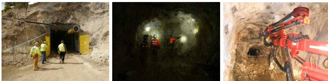
Figures 2 to 4: Mine Development at New Departure
