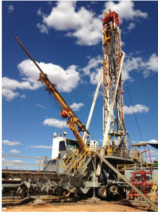
Ensign Rig 48 Development Drilling Utopia Field
