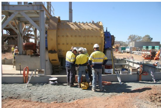
Wonawinta Silver Mine – Ball mill installation, 7 th May 2013
