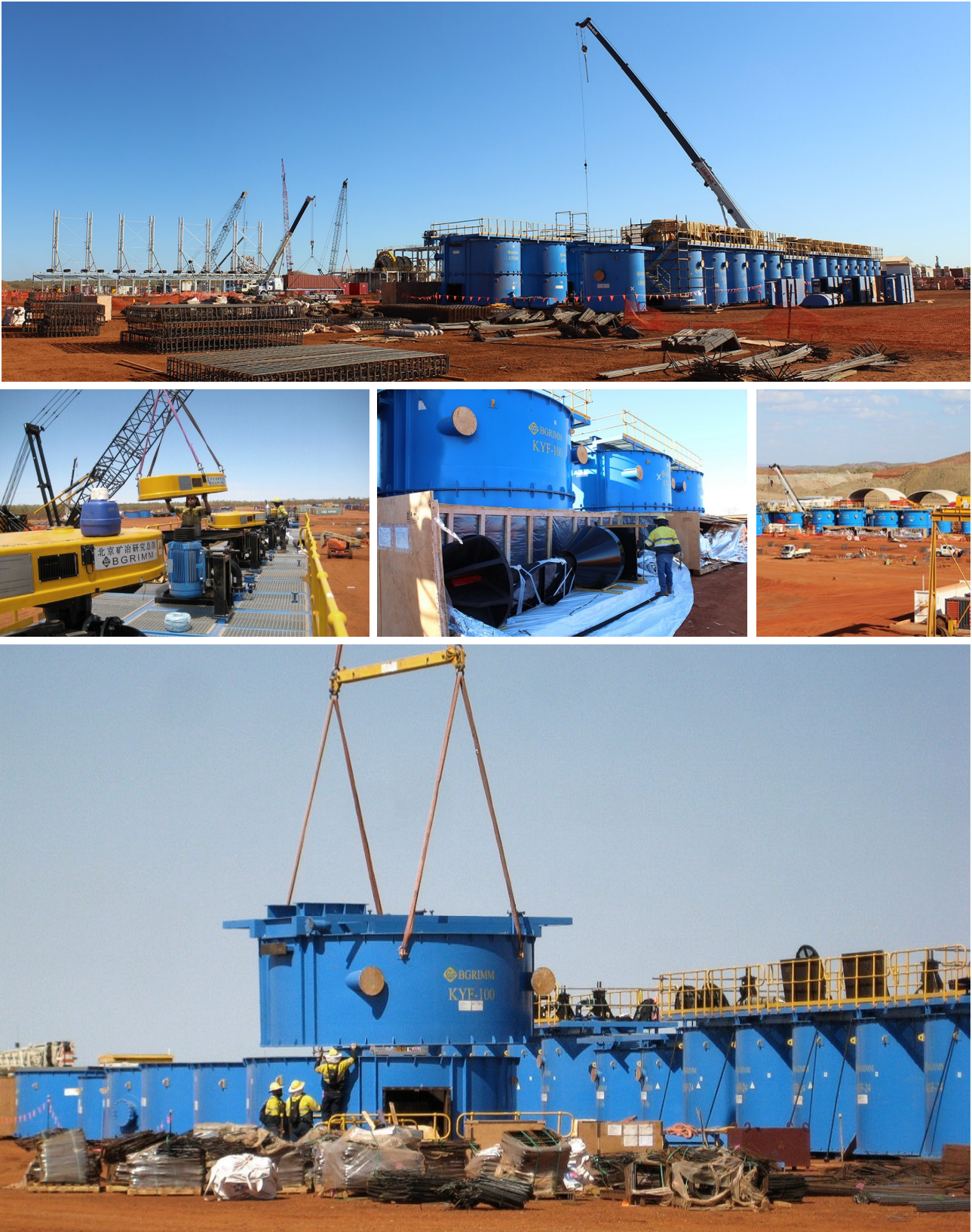
Figure 21: Flotation Cells being assembled...see Figure 7 for location details
