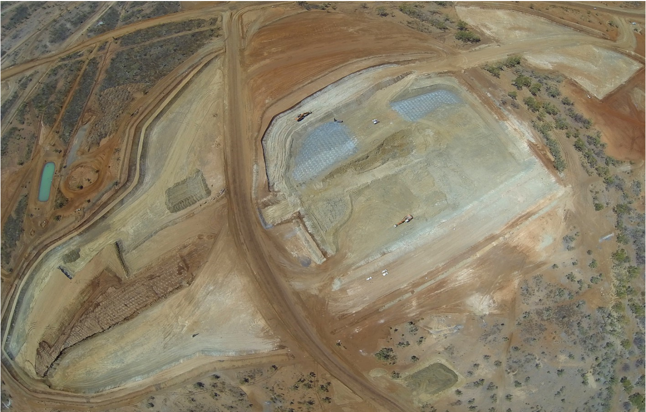
Figure 35: Aerial view over the LM Open-cut and Stage-1 DSO Pit. Ore blasted and remaining in-situ can be seen in the middle of the pit to the left, and mining is underway at the LM Stage-1 DSO Pit (centre right)...see Figure 7 for location details
