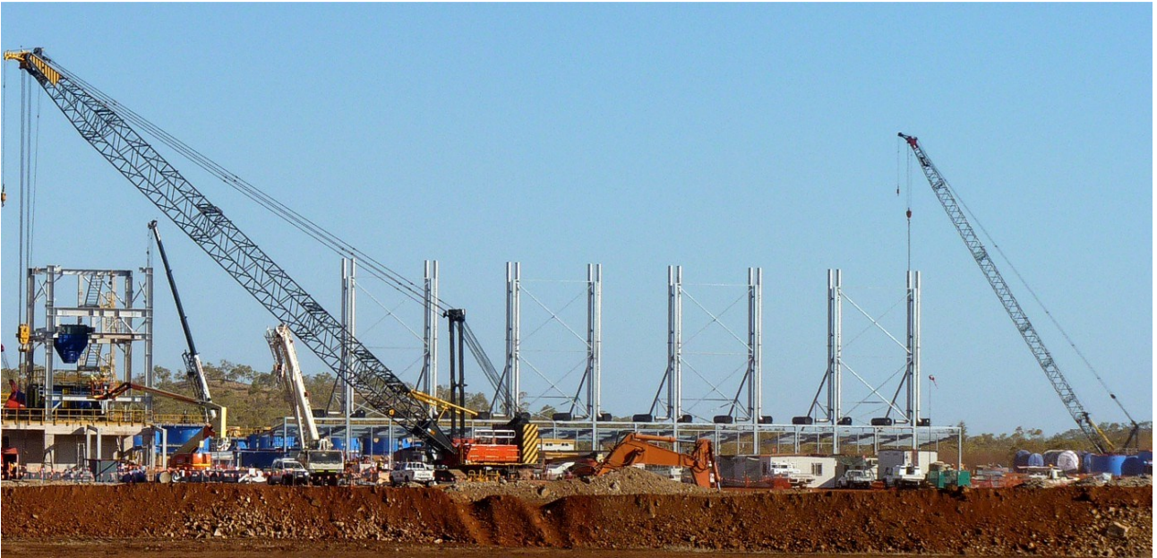
Figure 11: Power Station structural framework being erected...see Figure 7 for location details
