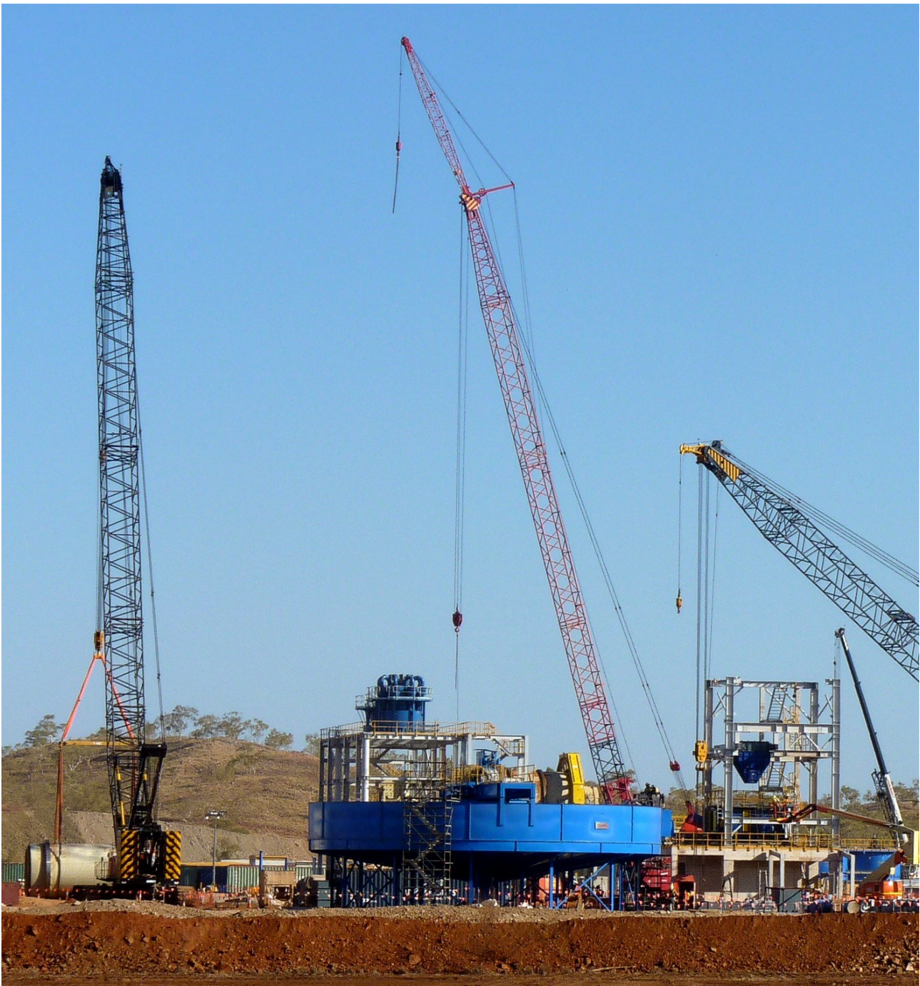
Figure 16: ...Tails Thickener in foreground, surrounded by large heavy lift Walz cranes. In background from left to right; De-agglomerator; Ball Mill and; HPGR...see Figure 7 for location details
