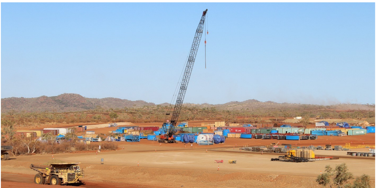
Figure 31: Lay-down area for process Plant component deliveries...see Figure 7 for location details
