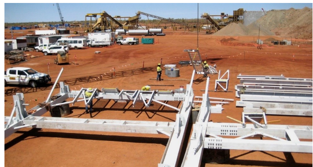
Figure 28: De-agglomerator foundations (left) and Power Station structural steel being assembled for tilt-up erection (right)...see Figure 7 for location details
