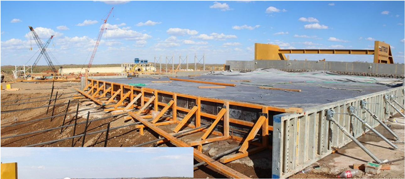
Figure 27: ROM slab poured and curing (above) and setting of reinforcing bars (left)...see Figure 7 for location details
