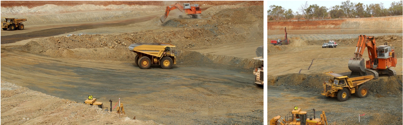
Figure 39: Dark ore zones are easily distinguished from waste in the LM Stage-1 DSO Pit
