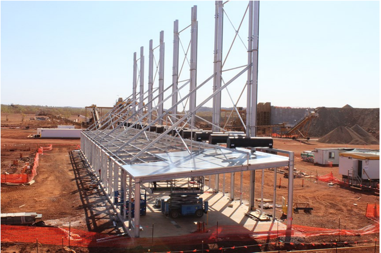
Figure 22: Construction of the Power Station...see Figure 7 for location details
