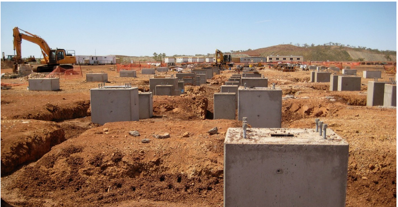
Figure 23: Gravity Jig foundations...see Figure 7 for location details
