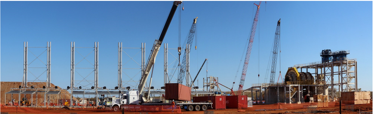
Figure 3: Power Station (left) and Ball Mill (right)...see Figure 7 for location details
