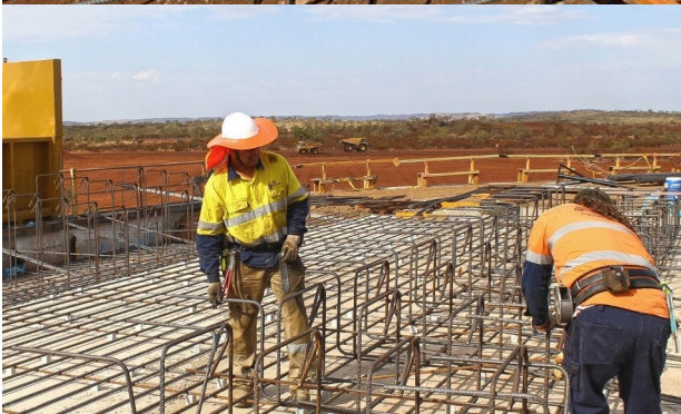
Figure 27: ROM slab poured and curing (above) and setting of reinforcing bars (left)...see Figure 7 for location details
