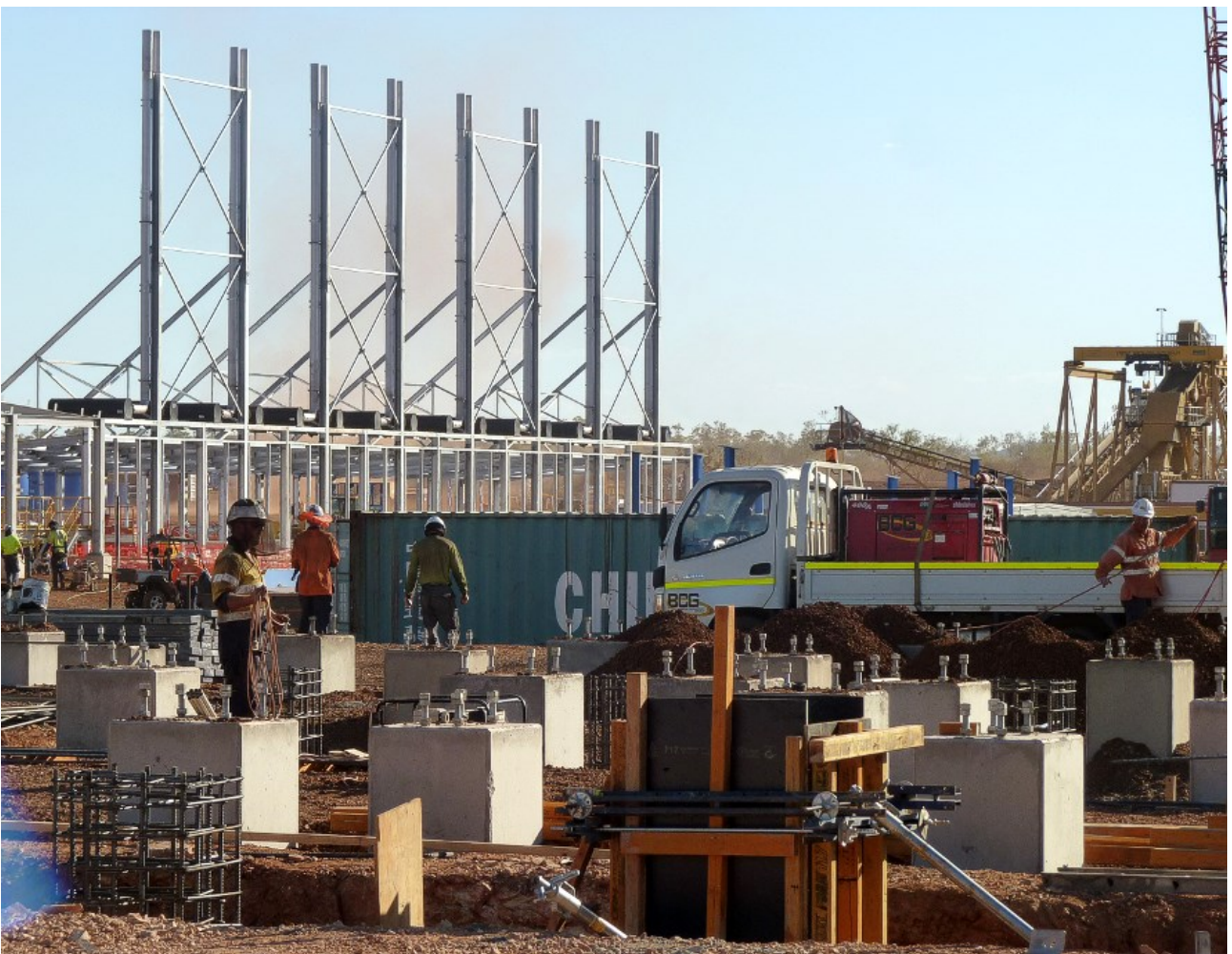
Figure 26: De-agglomerator foundations (foreground) and Power Station (background)...see Figure 7 for location details
