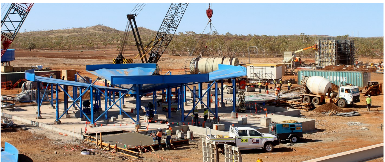
Figure 20: Assembly of the Gravity Thickener...see Figure 7 for location details
