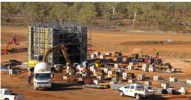
Figure 28: De-agglomerator foundations (left) and Power Station structural steel being assembled for tilt-up erection (right)...see Figure 7 for location details
