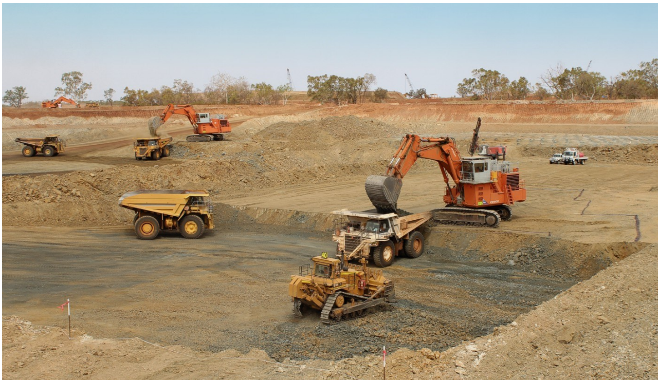
Figure 32: Mining at LM Stage-1 DSO Pit...see Figure 7 for location details
