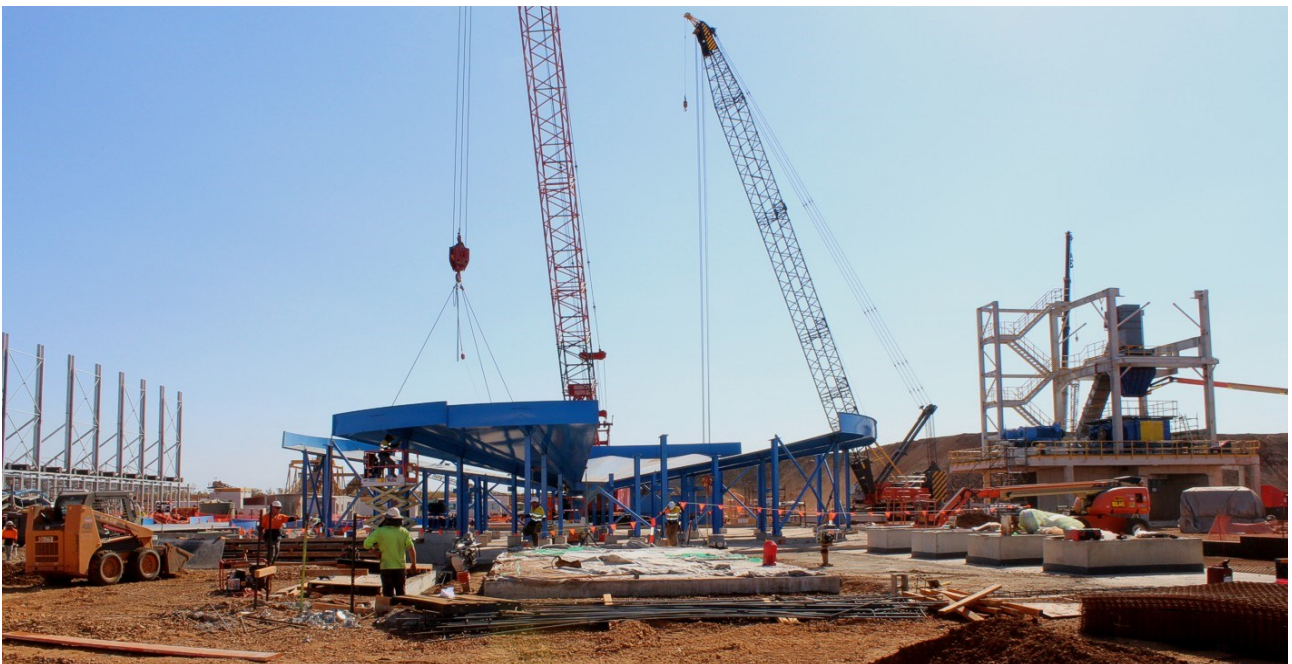
Figure 19: Assembly of the Gravity Thickener...see Figure 7 for location details
