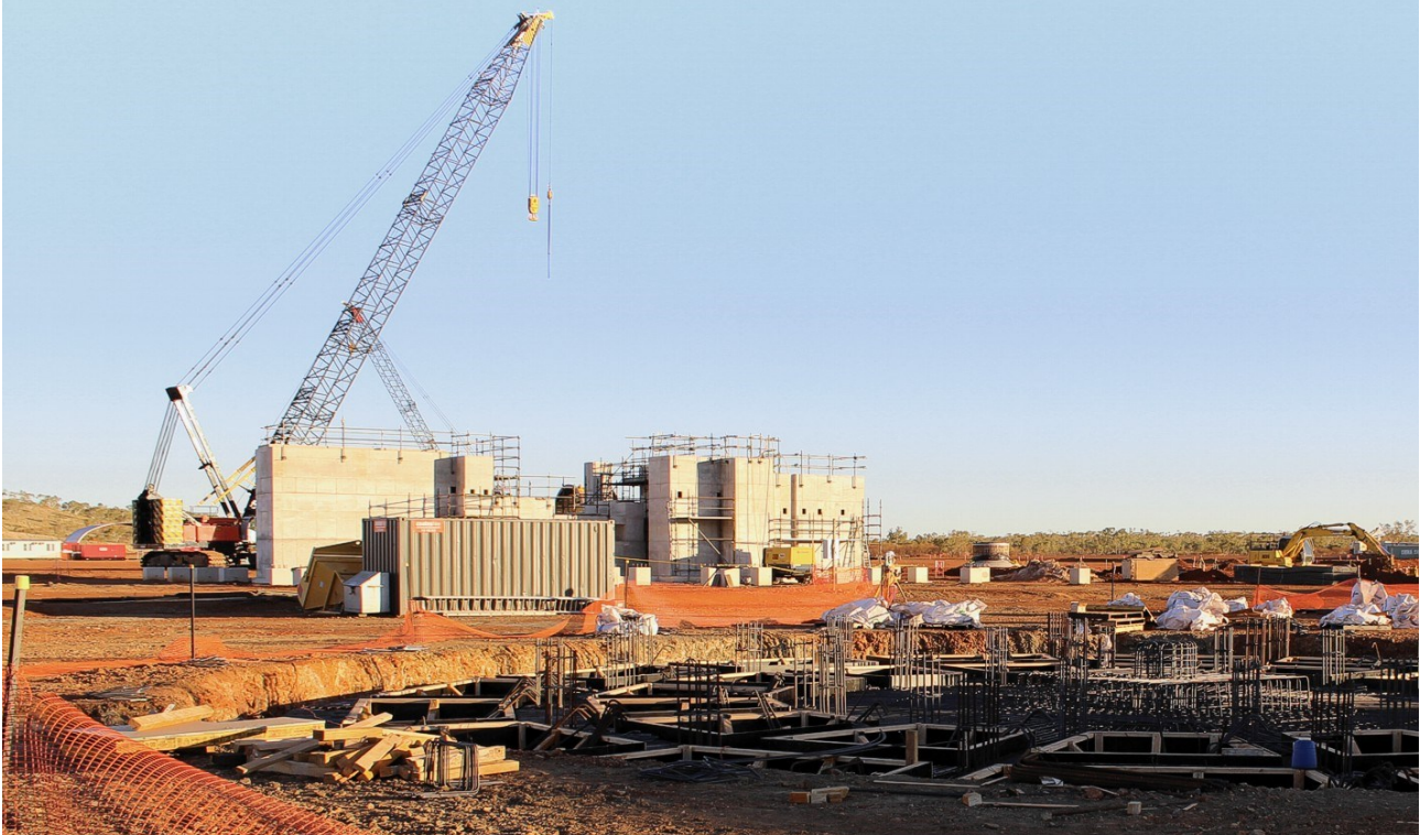
Figure 1: Formwork for gravity thickener in foreground, and completed concrete work at Ball Mill housing in background.
