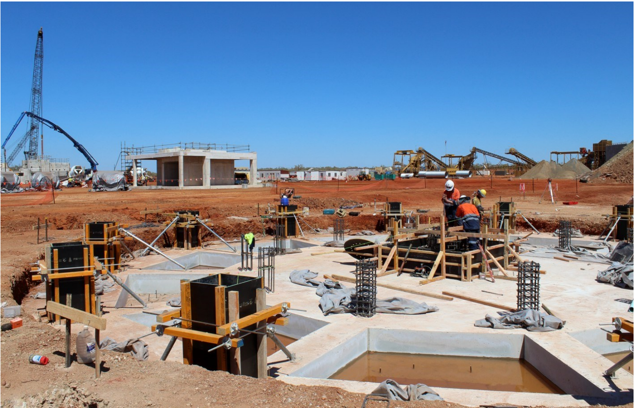
Figure 3: Foundations for the tailings thickener.
