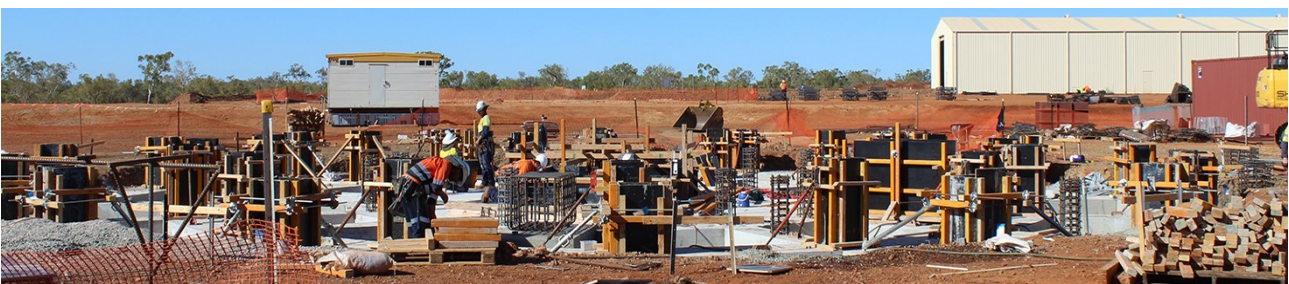
Figure 5: Activity during the concrete pour of foundations at the gravity thickener
