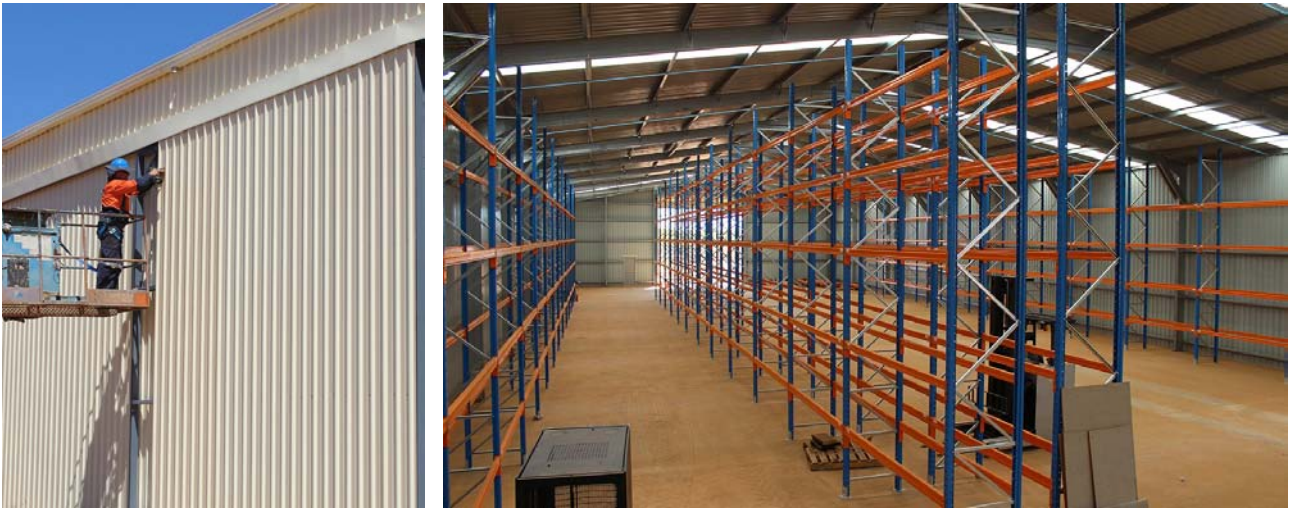
Figure 15: Final touches to the new Stores Warehouse, which also includes a data centre and offices
