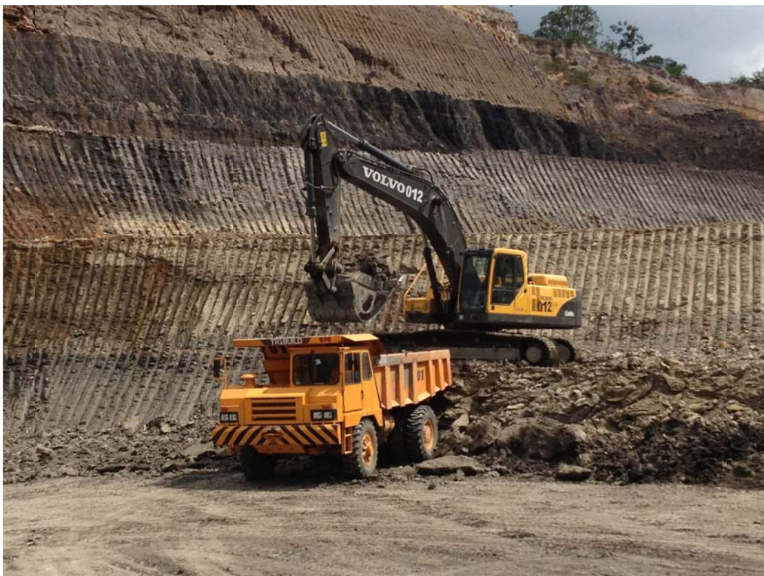
Figure 2: Photograph showing waste being loaded onto one of the new TRXBUILD D20 dump trucks.
