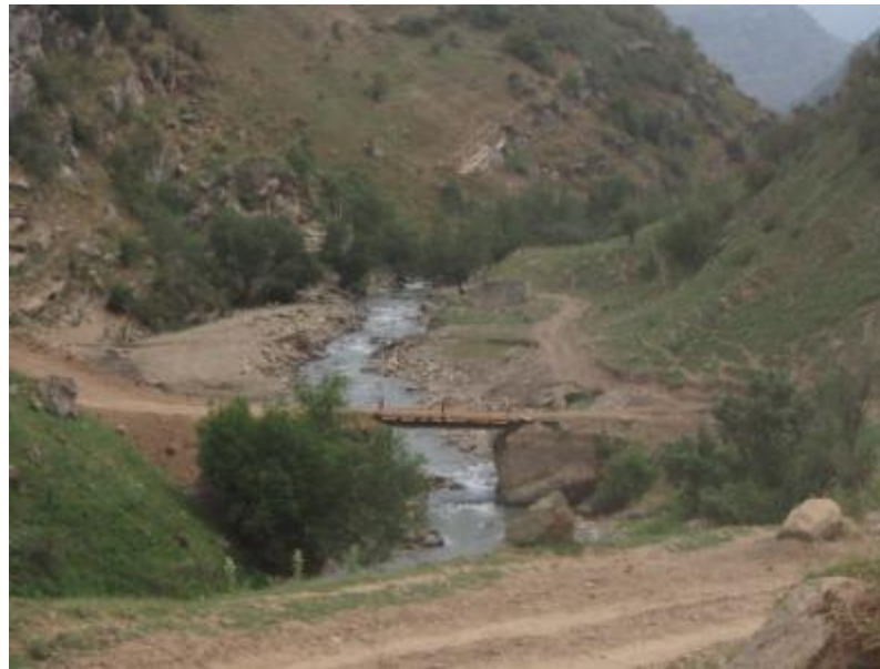
Recently constructed bridge over the Kargasha River
