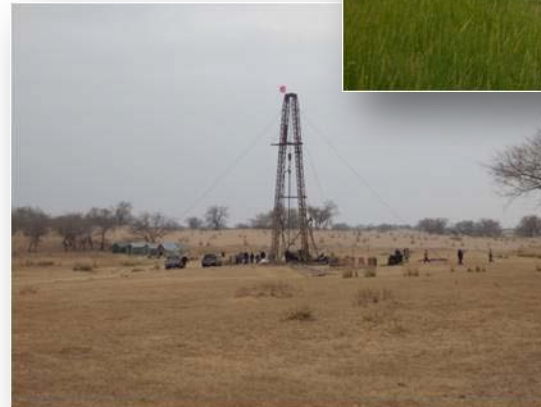
Drill Rig on Inner Mongolia Site
