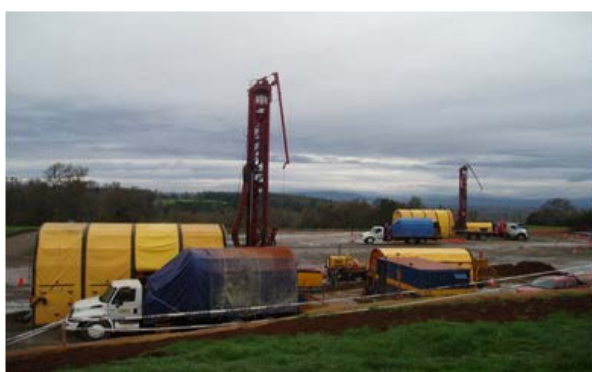
Monitoring Well Drilling on Vertical Drilling Pad
