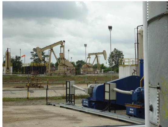
Figure 1 - Water injection equipment onsite at the WBEXT water flood project
