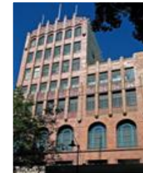
299 Bourke Street (Men's Store) Melbourne
