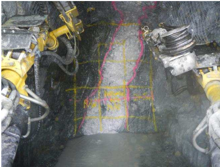
1400 Level North Ore Drive
