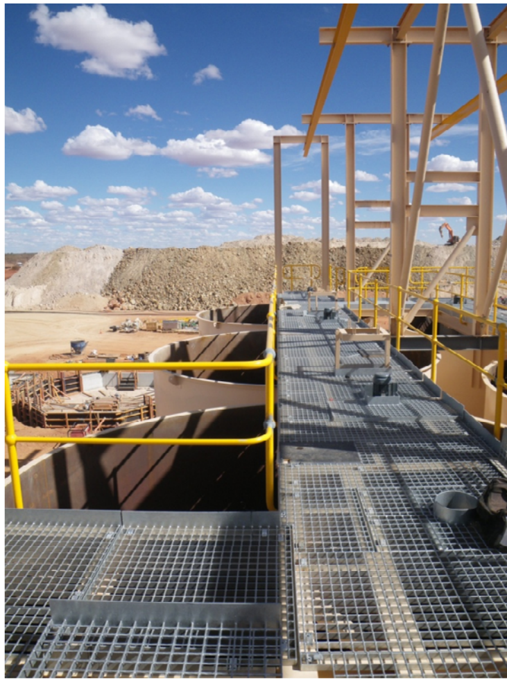
Figure 3. Access way on top of leach tanks, looking towards ROM pad.
