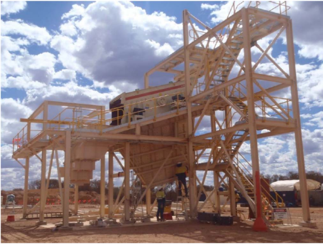
Figure 5. Crusher screening deck installed
