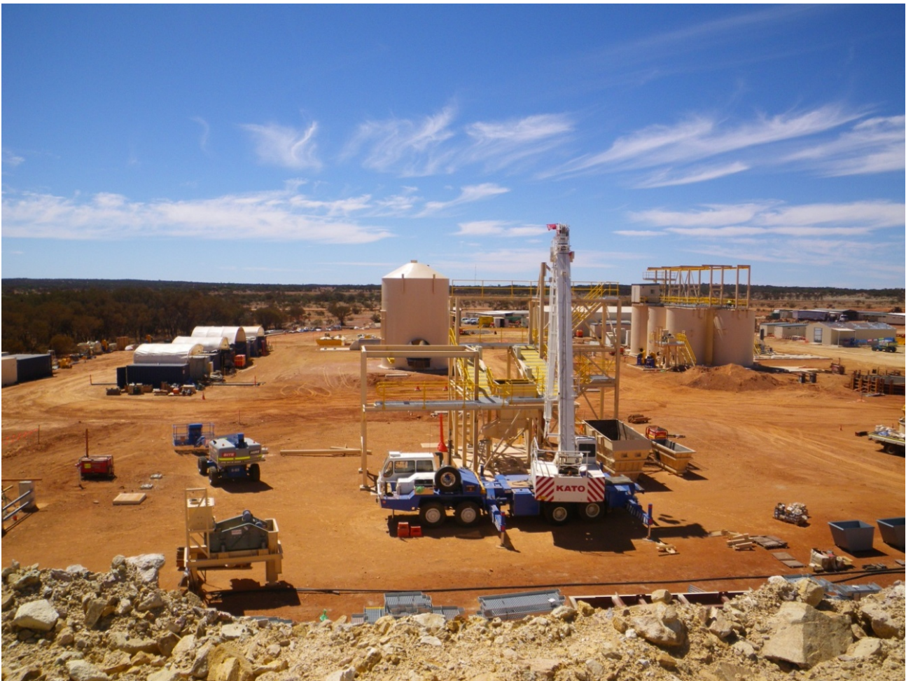
Figure 2. Overview of processing plant site showing construction progress.
