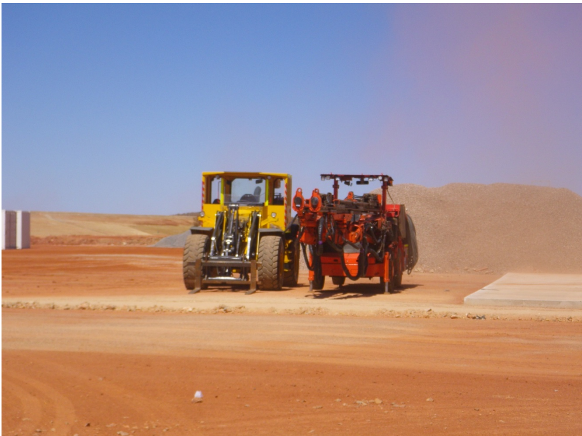
Figure 8. First items of underground mining contractor's fleet delivered to site.
