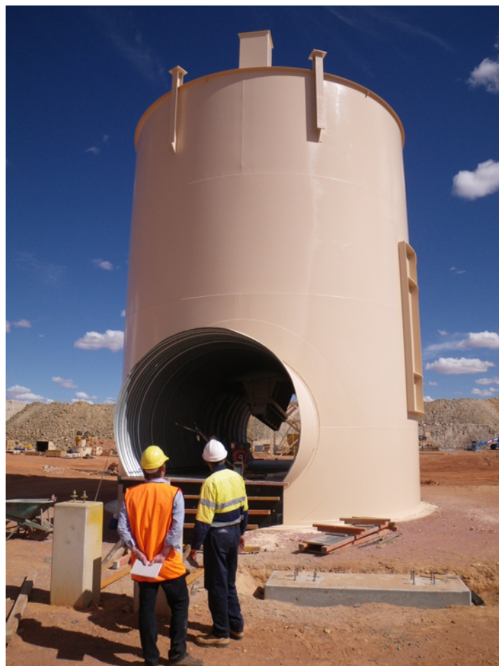
Figure 4. Completed fine ore bin with conveyor tunnel.
