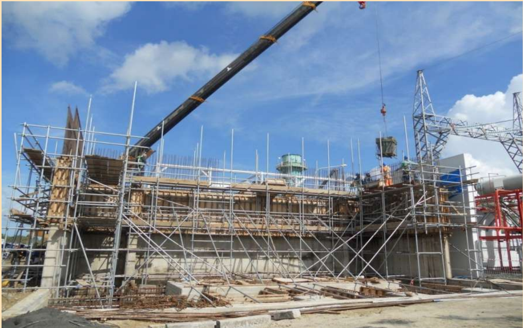
Pouring concrete for Blast Wall ST-28 Main Transformer
