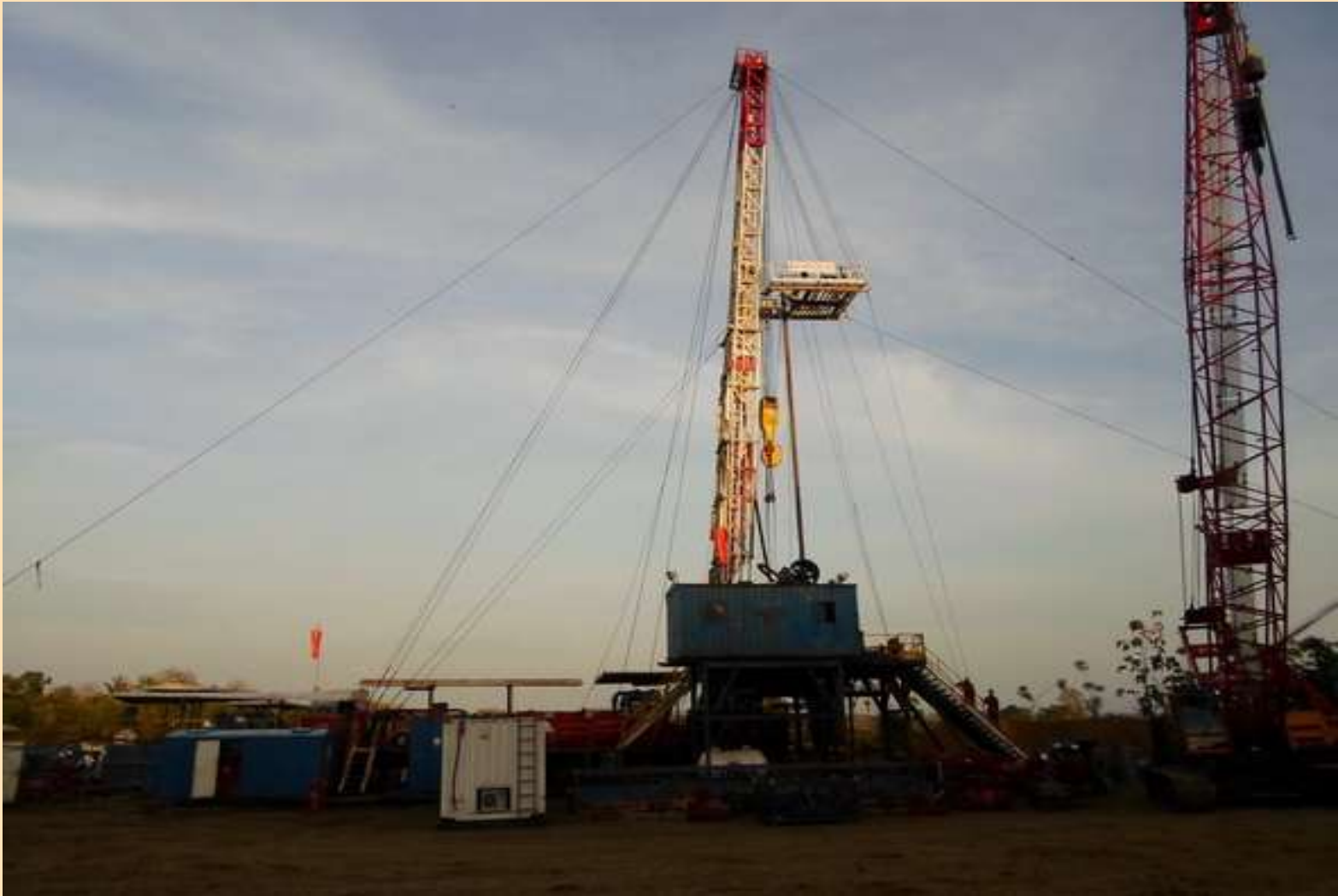
Rig Mast & Substructure for Walanga #3
