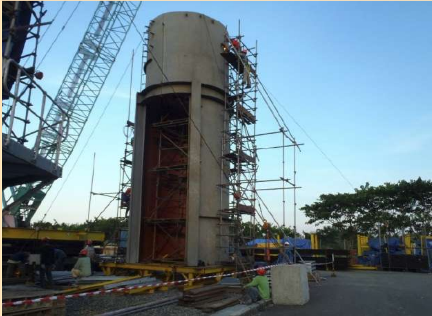
Install Scaffold Stack Tier 2
