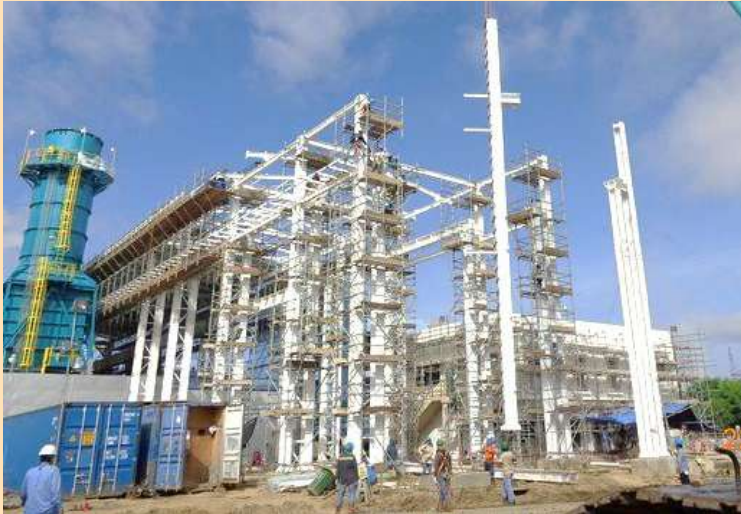
Erection Install Column for OTC
