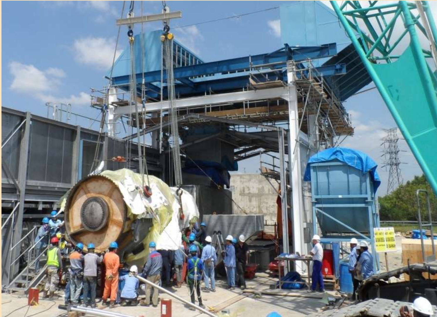
Installation of Gas Turbine
