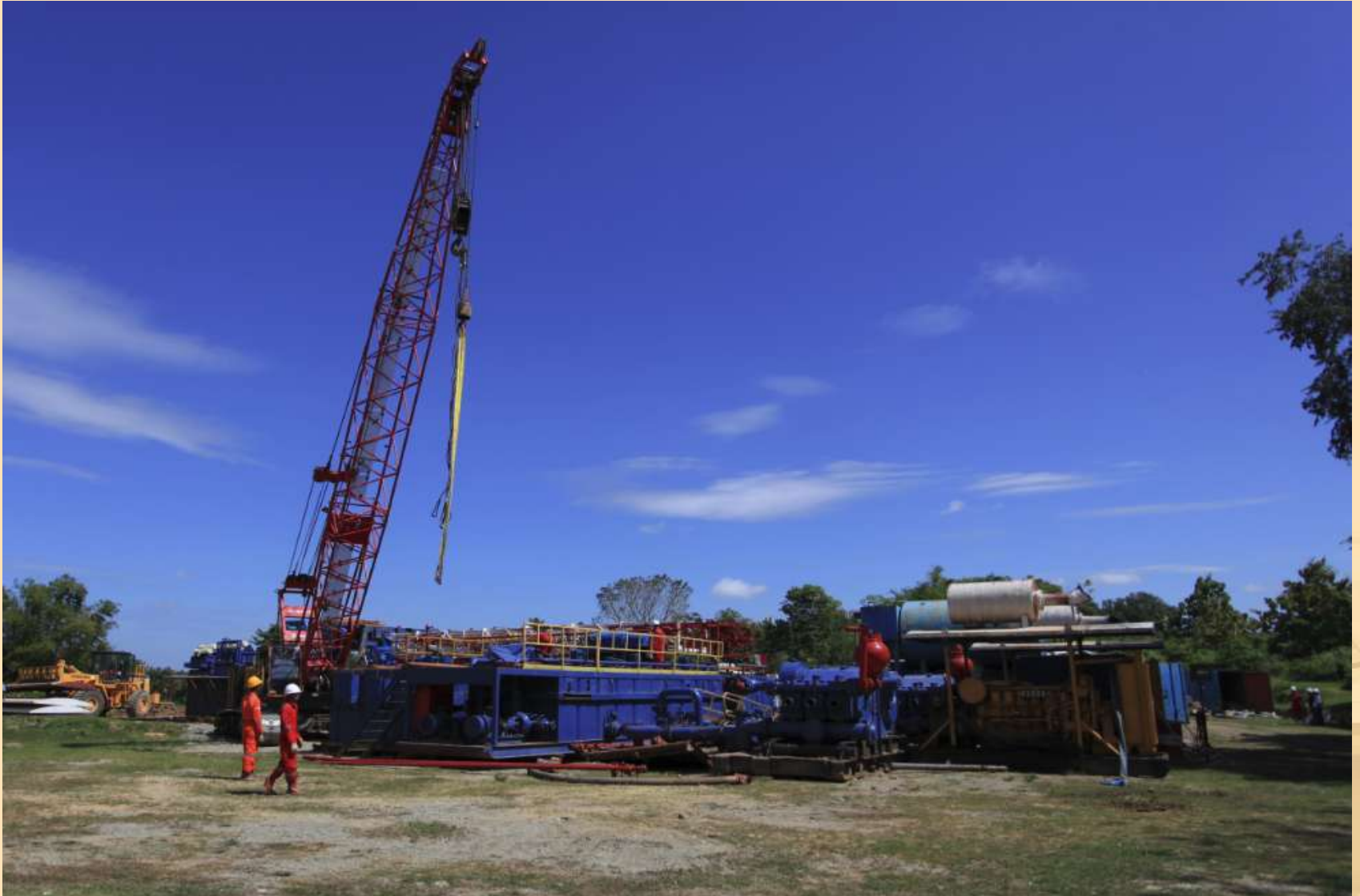
Preparation for drilling activities for Walanga #2 at Wasambo Gas Field
