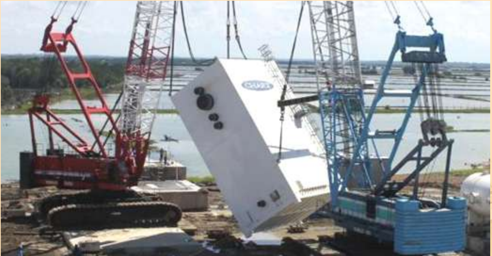
Crane 1 taking the full load, Crane 2 turning Cold Box to position
