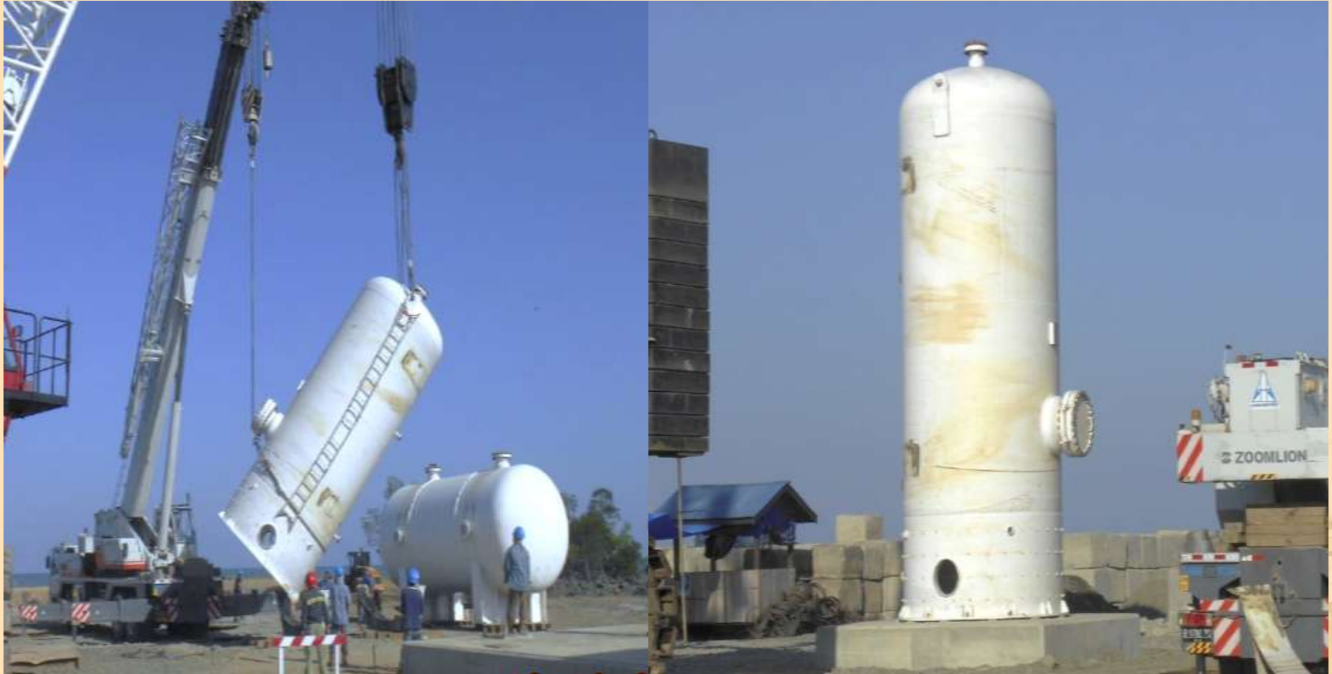
Erection the MR Vapor Surge Drum D-2206 to fix foundation
