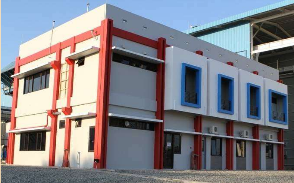
Central Control Room and Office Building
