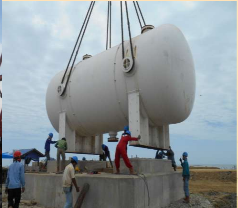
Erection the MR Accumulator Drum D-2205 to fix foundation
