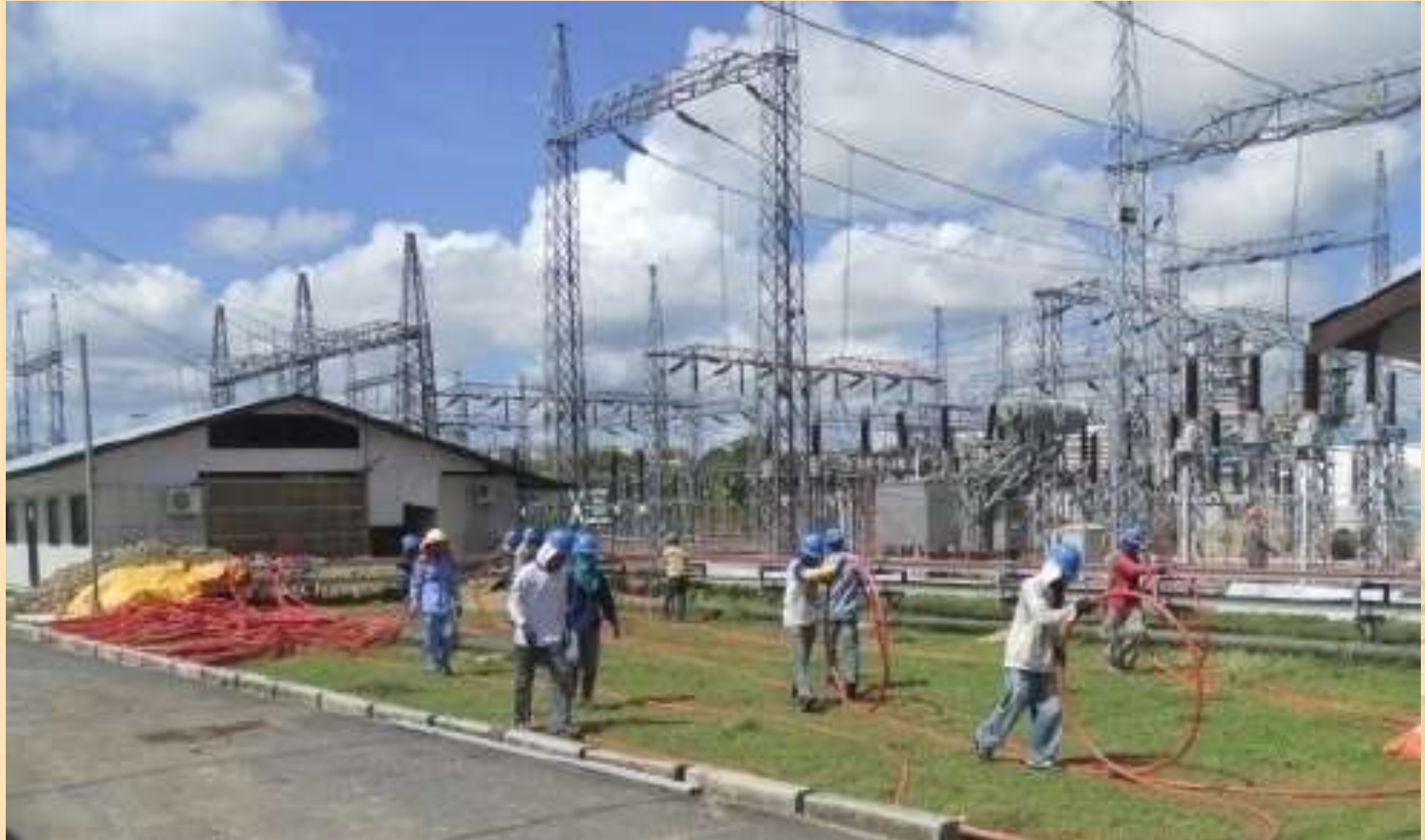
Pulling Cable from GT21 to GT22
