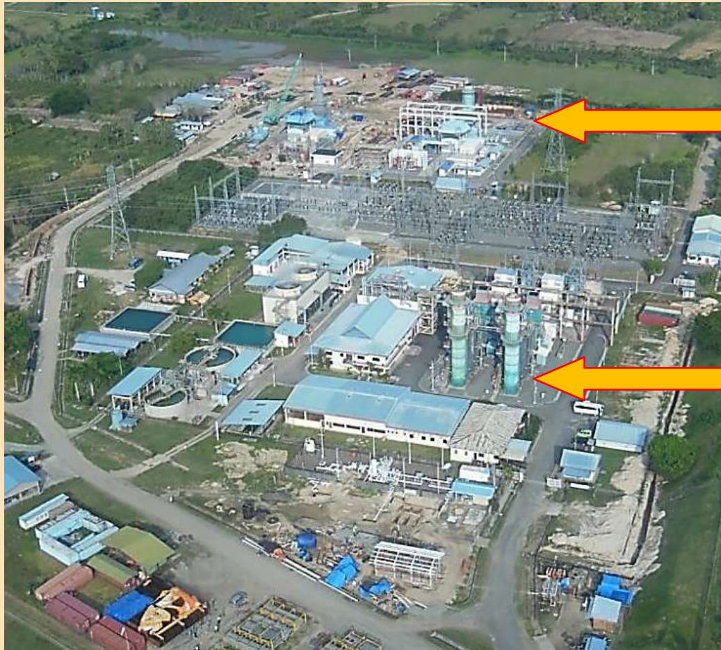
Aerial view of Sengkang Power Plant
