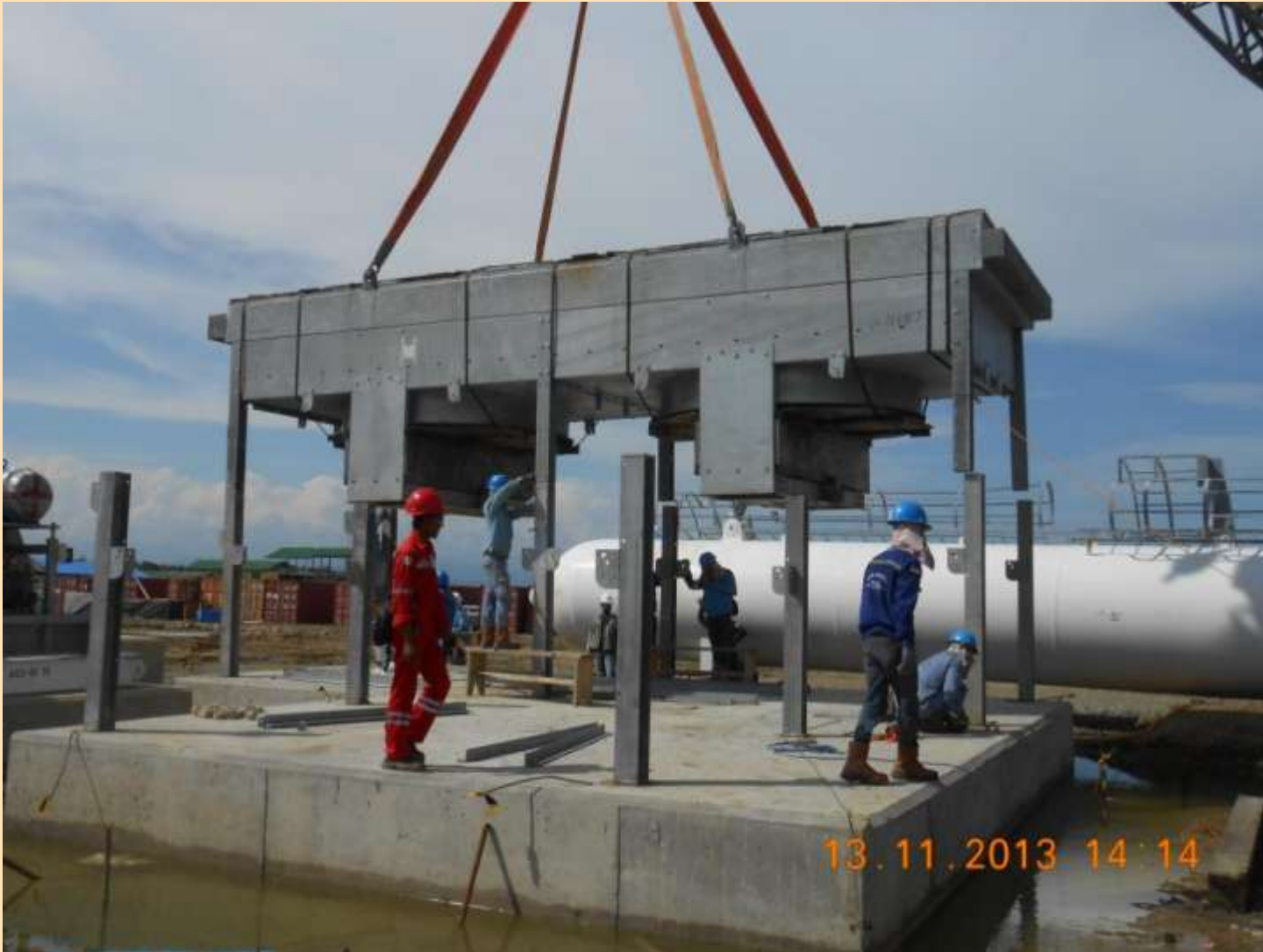
Erection Treated Gas & Lean Amine Cooler: Column installation in progress
