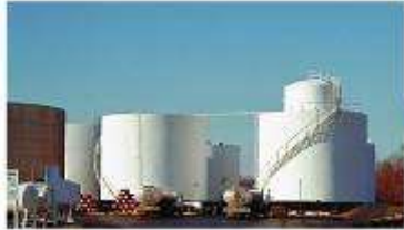
Diesel Fuel Storage at Refinery
