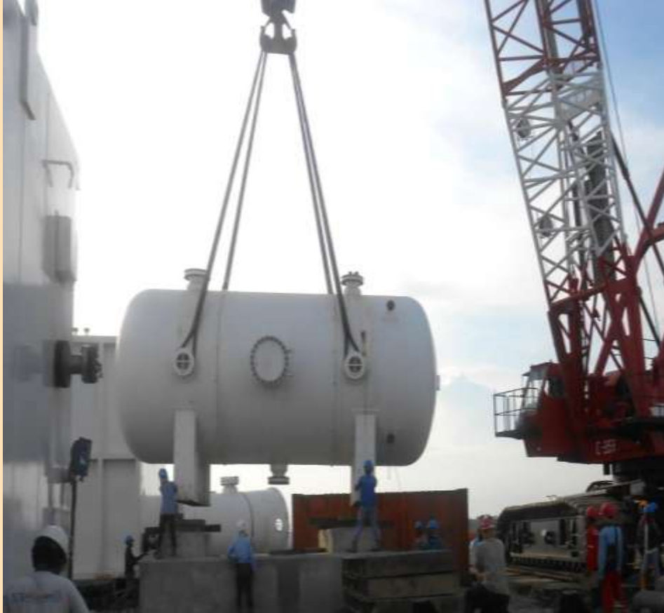
Erection the MR Accumulator Drum D-2205 to fix foundation
