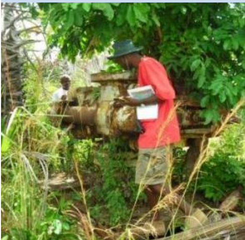
Locating the Kipini-1 wellhead
