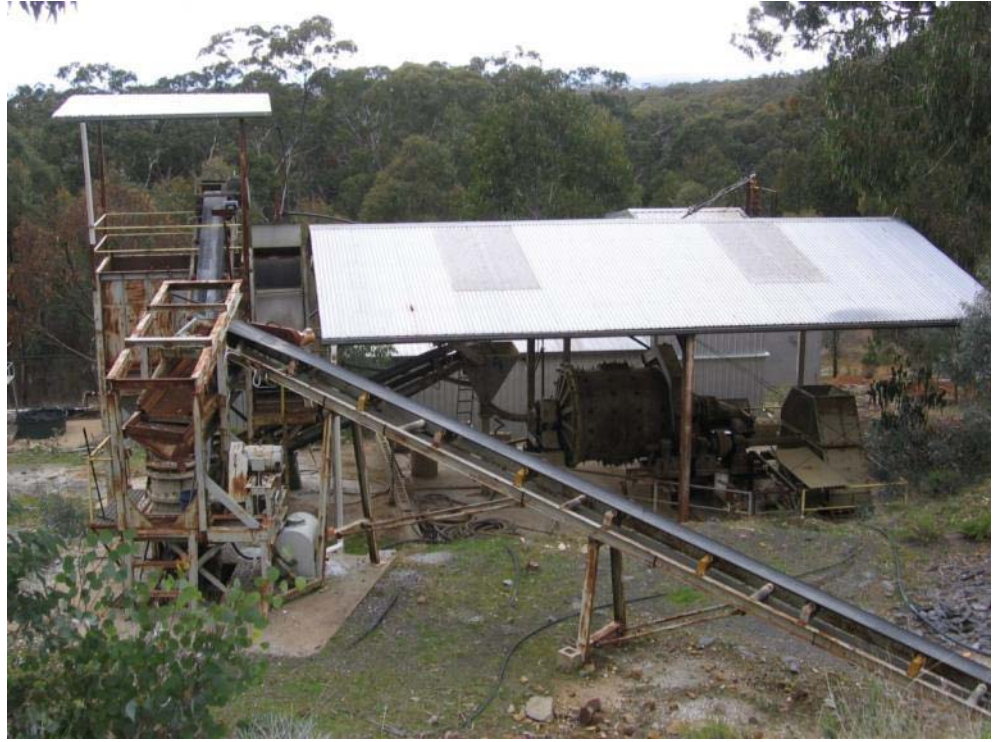
Fiddlers Ck Crushing circuit, Ball Mill – concentration circuit in background
