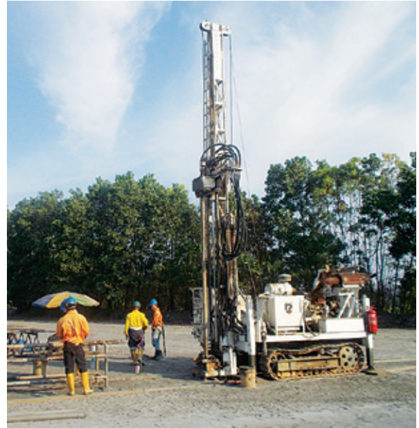
Drilling of tailings dam at Lubuk Mandi in Malaysia.
