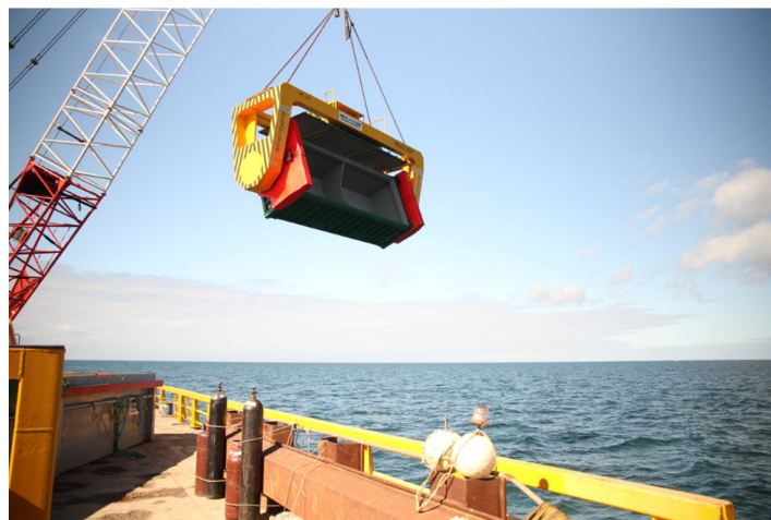
Container being rotated, delivering ore to “ship’s hold”
