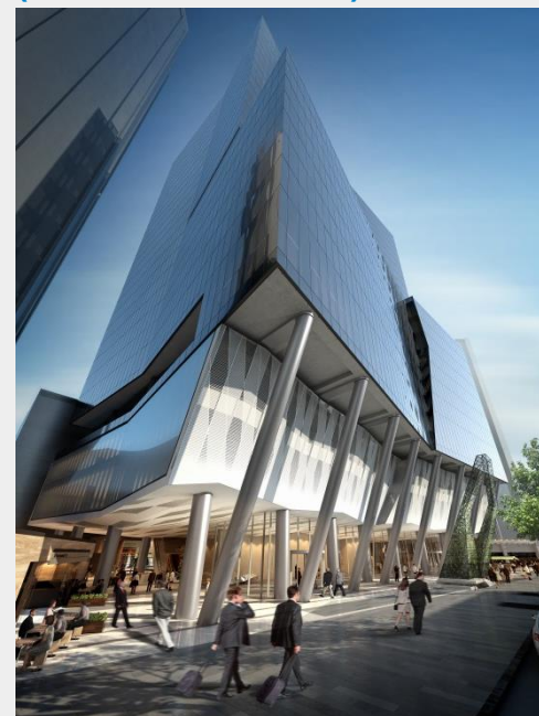
567 Collins Street, Melbourne (under construction)
