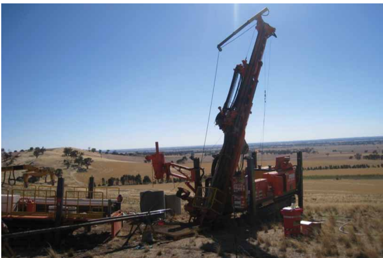
Figure 3 – Drilling geotechnical hole GTC2 at Golden Camel
