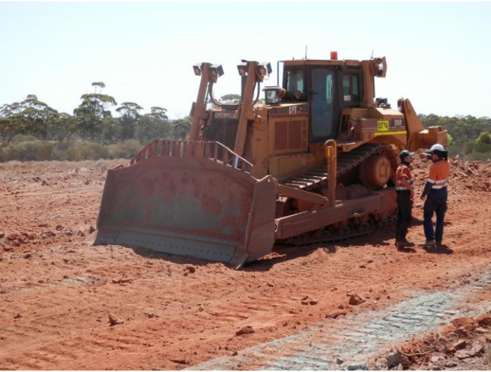
Image 4: Vegetation and top soil clearing
