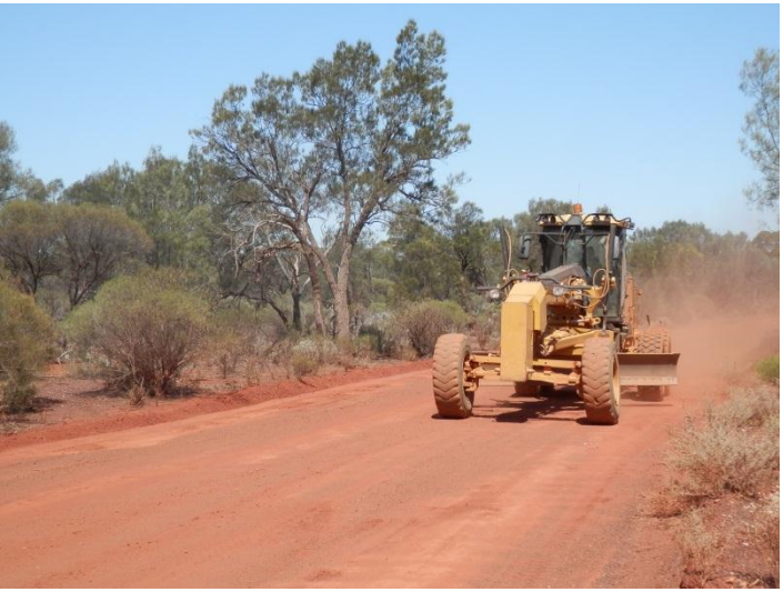
Image 5: Haul road construction
