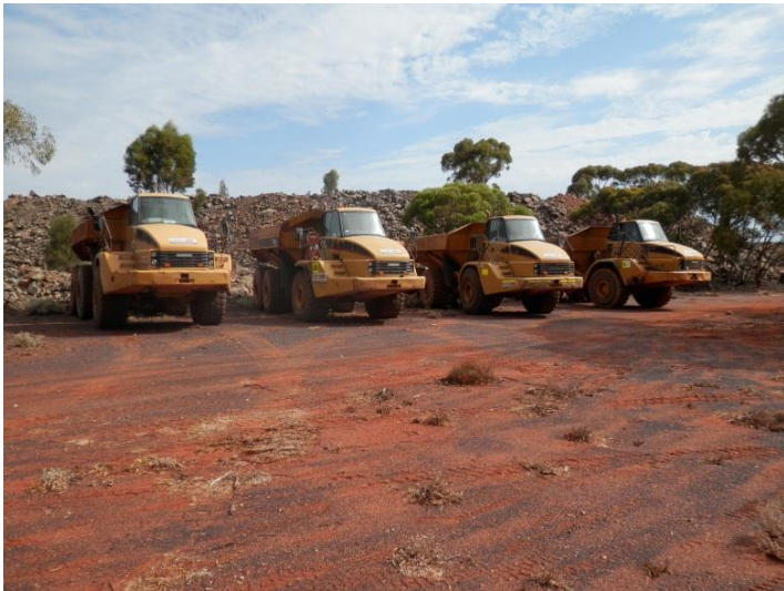
Image 2: Contractor haul trucks delivered to site
