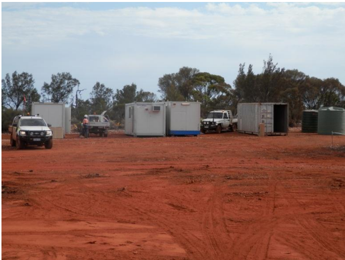
Image 3: Initial office and workshop facilities
