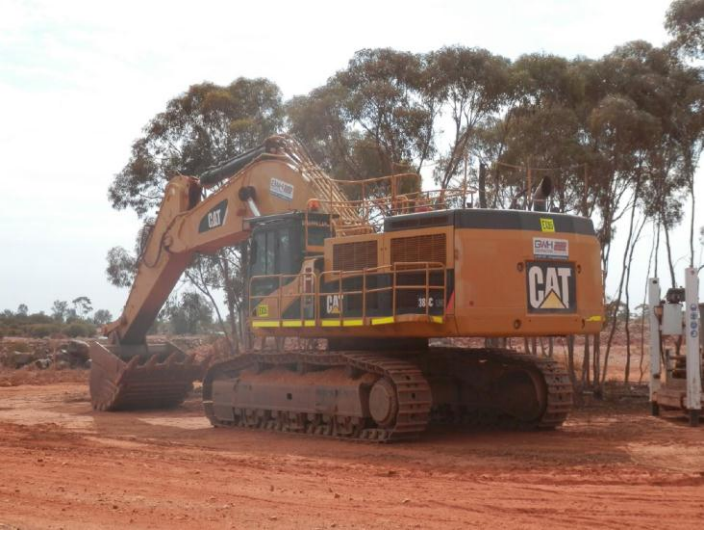
Image 6: Excavator on site
