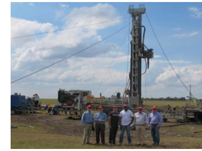
Pilot Test drilling
