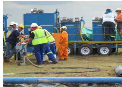
Pilot Test cement job crew
