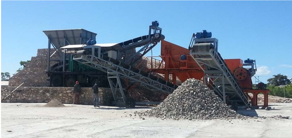
Dry Commissioning Kupang Process Plant - 30 Jun13
